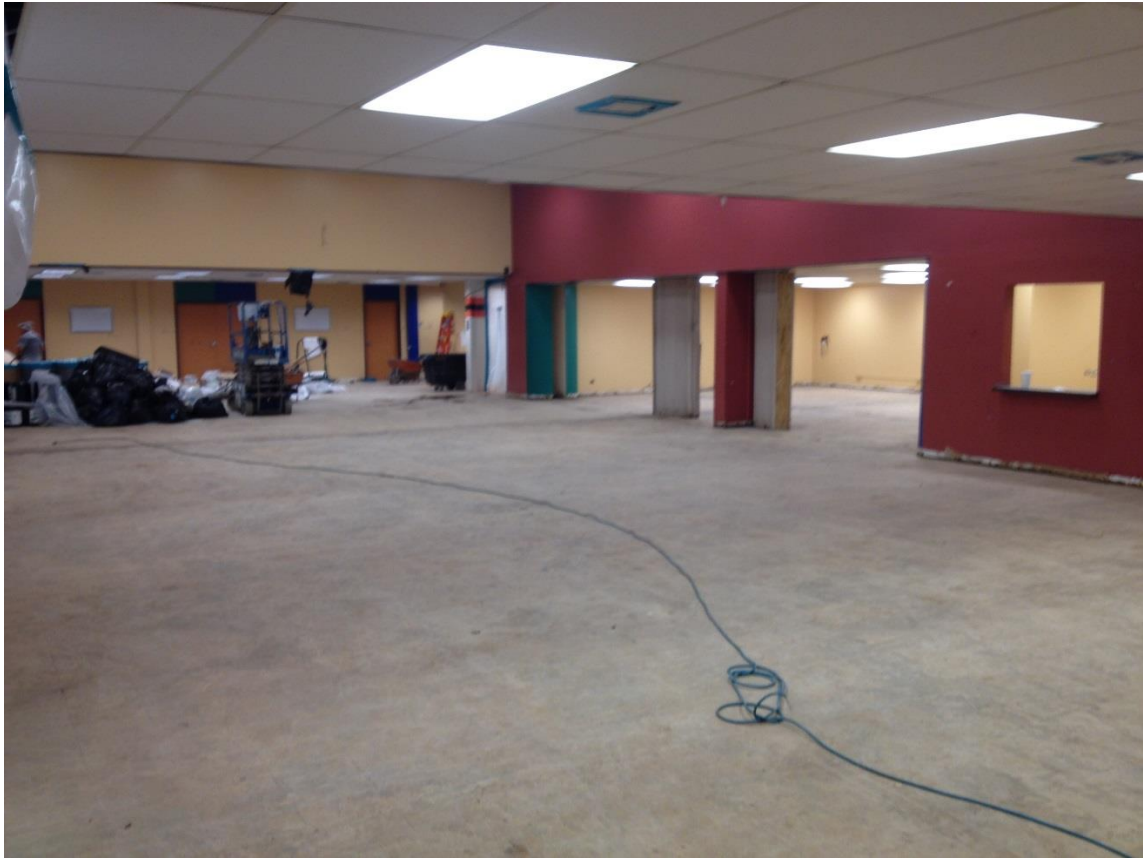
M.S. Stage/Cafeteria Remodel
