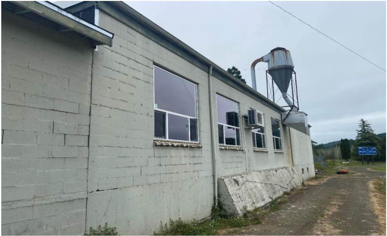
Photo 5: North Wing – Wood Shop – CMU Wall – Attempted Exterior Repair – Wall Physically Flexes with little effort of pushing. Inadequate supported mechanical equipment.
