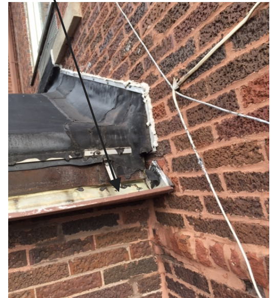
Gutter Damage
