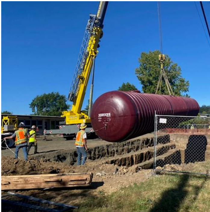
Fire Detention tank installed
