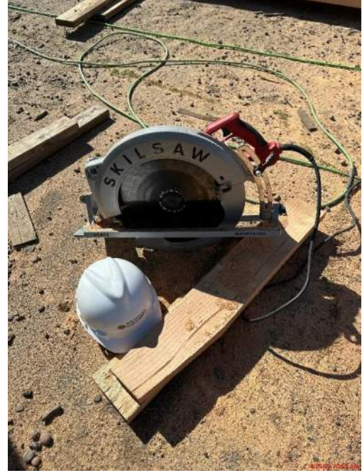
CHHS – One big saw (cutting large members)
