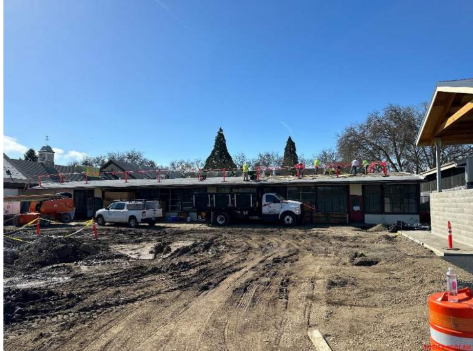
CHHS – B wing re-roofing
