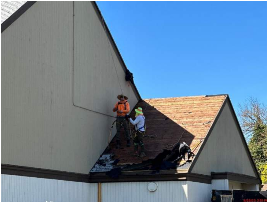
CHHS – Re-roofing Gym
