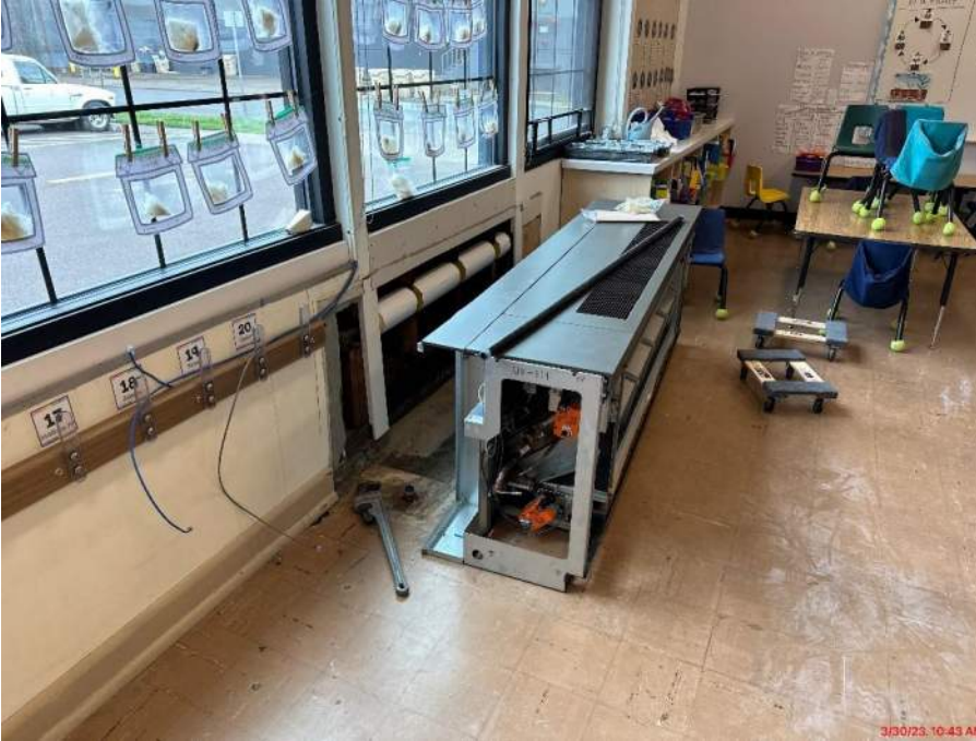
Franklin – Unit ventilator swap out
