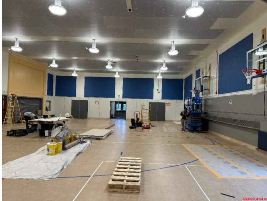
Franklin – Gym acoustical panels and FRL installing
