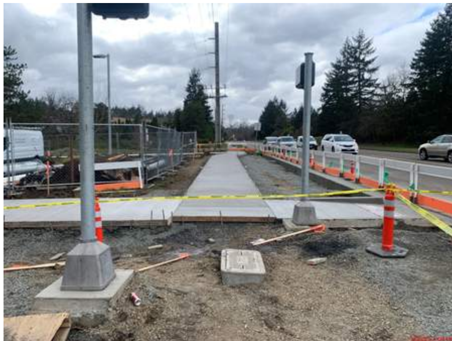
Aspen intersection work
