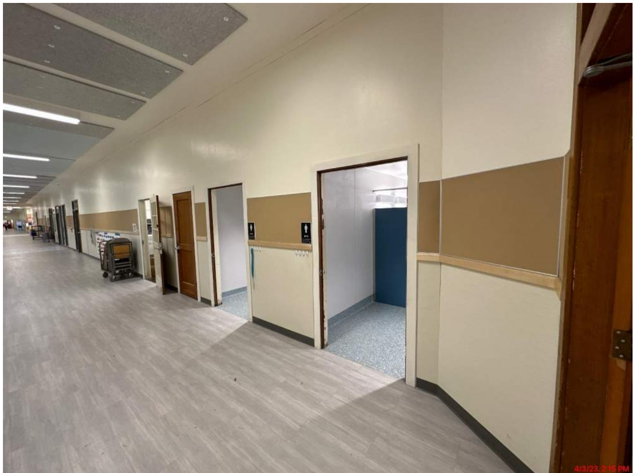
Franklin – Added tack board and chair rail west side of hallway
