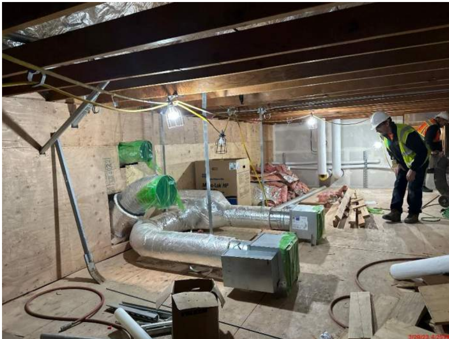
CHHS – misc. ductwork installation in attic space
