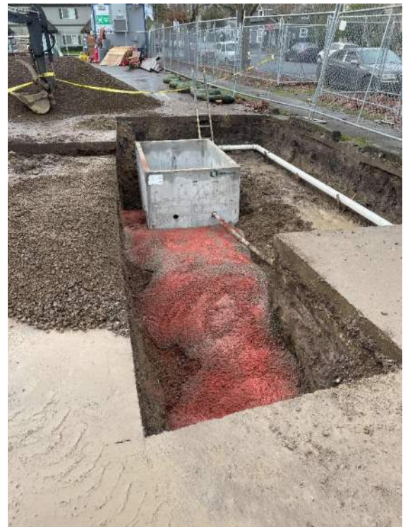
Franklin – New transformer underground and vault set
