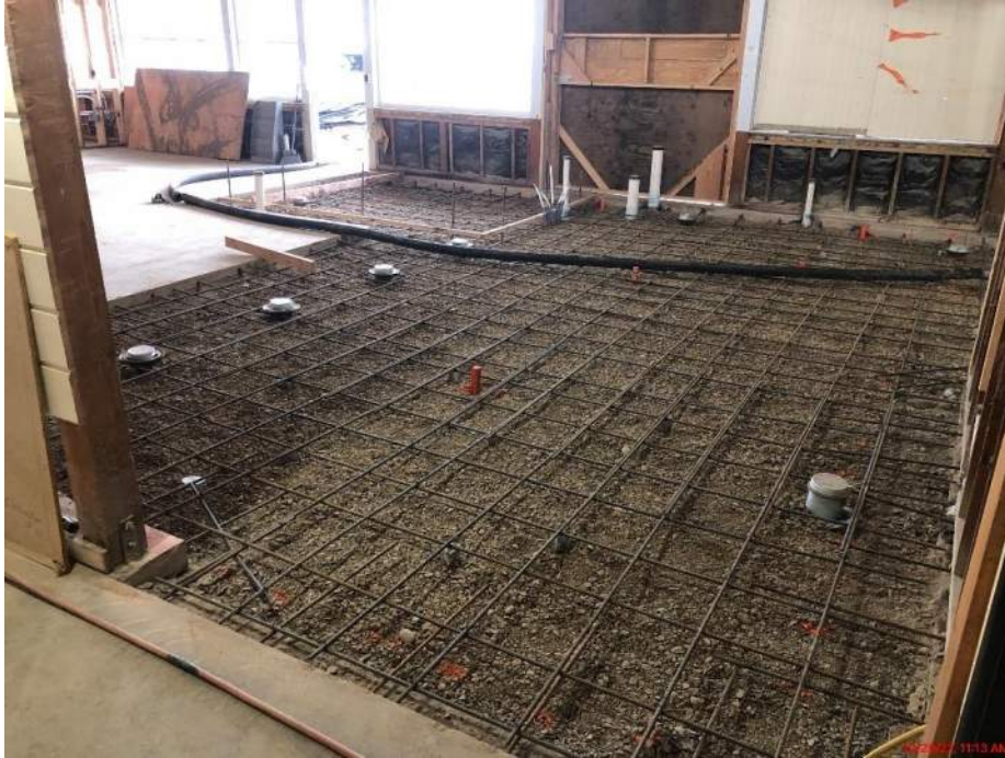
CHHS –New bathroom area slab prepped
