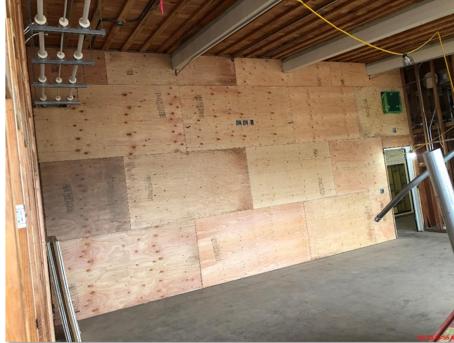
Shear Wall and other framing going up!
