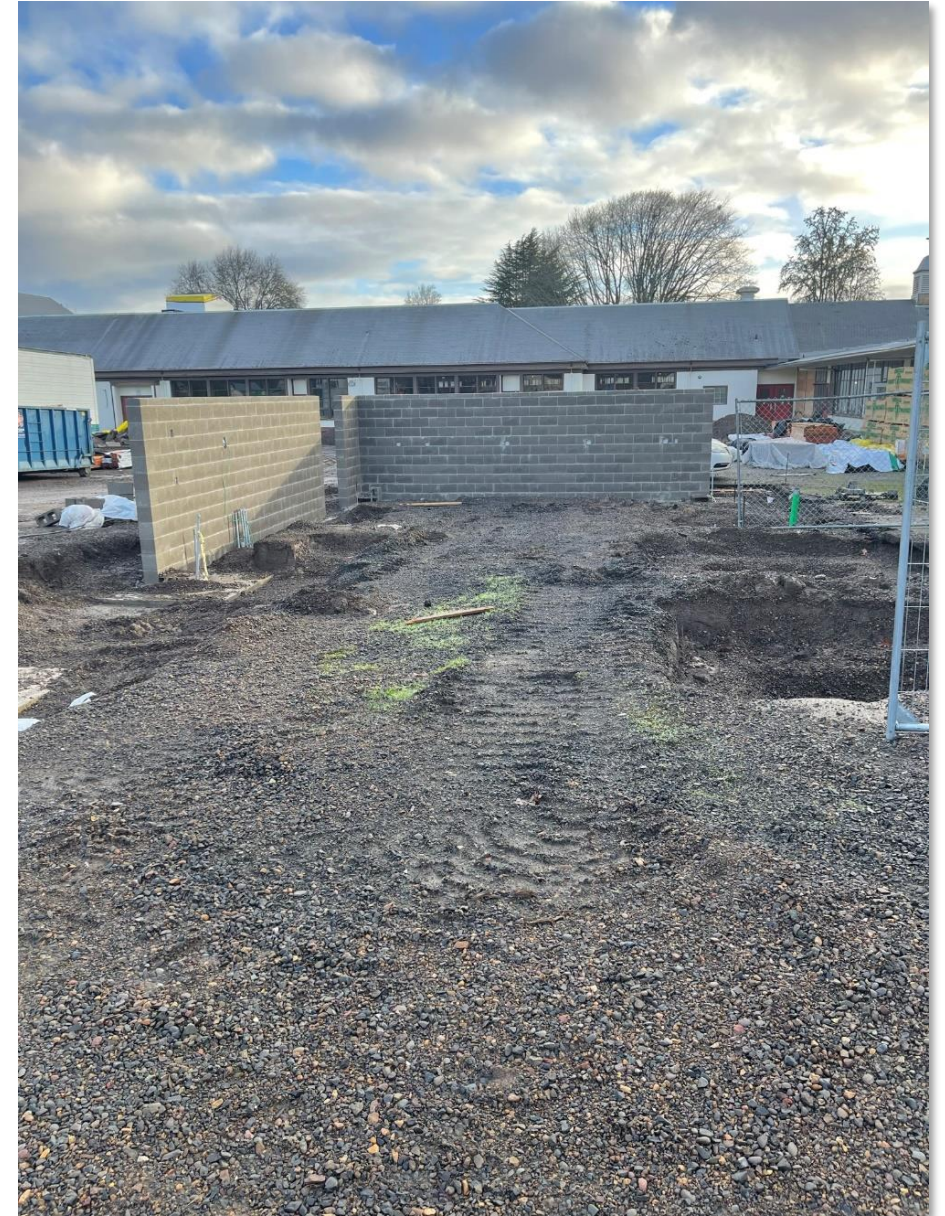
Covered Outdoor Learning progress
