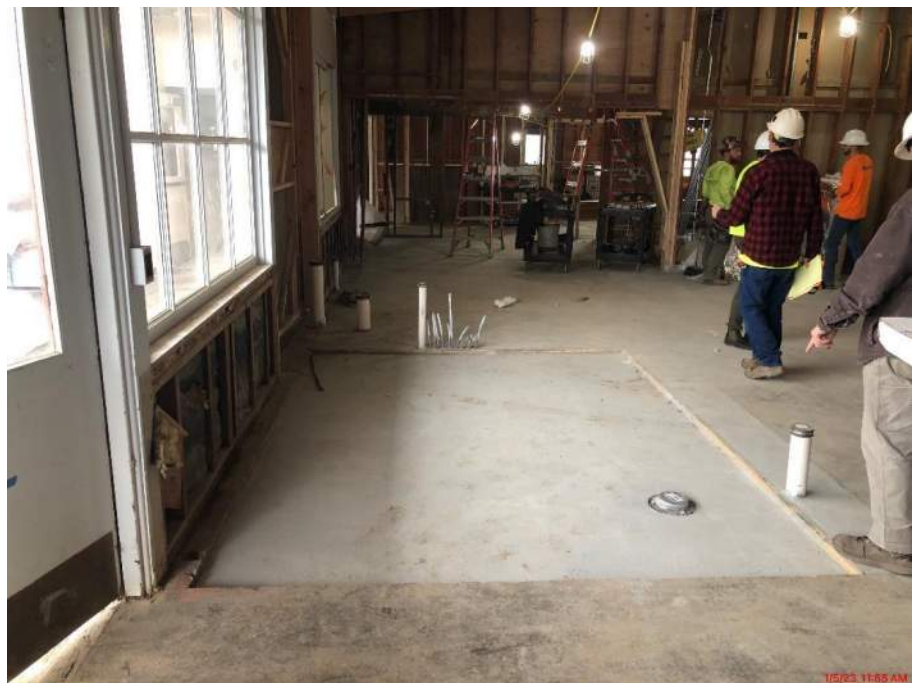
CHHS – New bathroom slab in place
