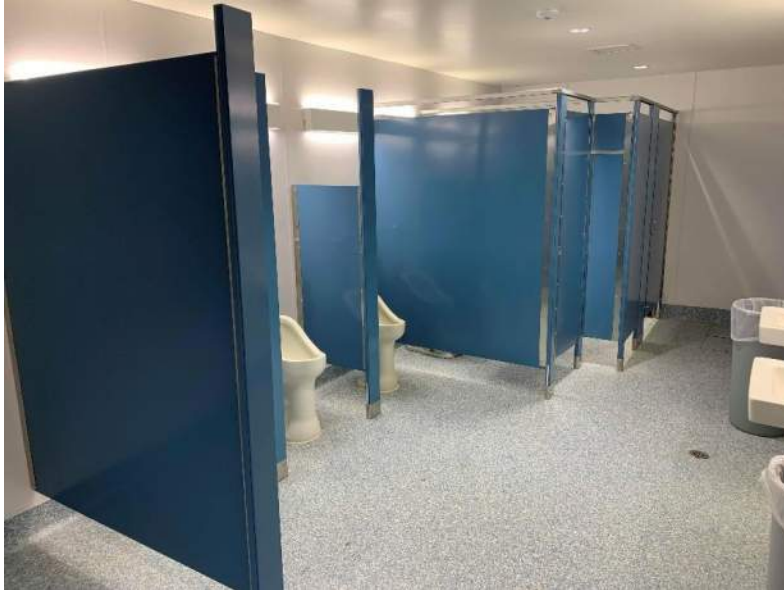
New toilet partitions in remodeled restroom areas
