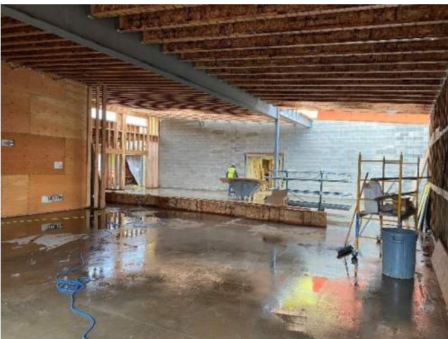
New Addition – Cafeteria
