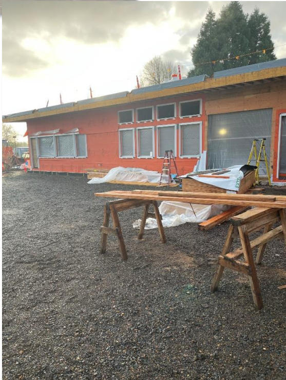
New Addition framing continues
