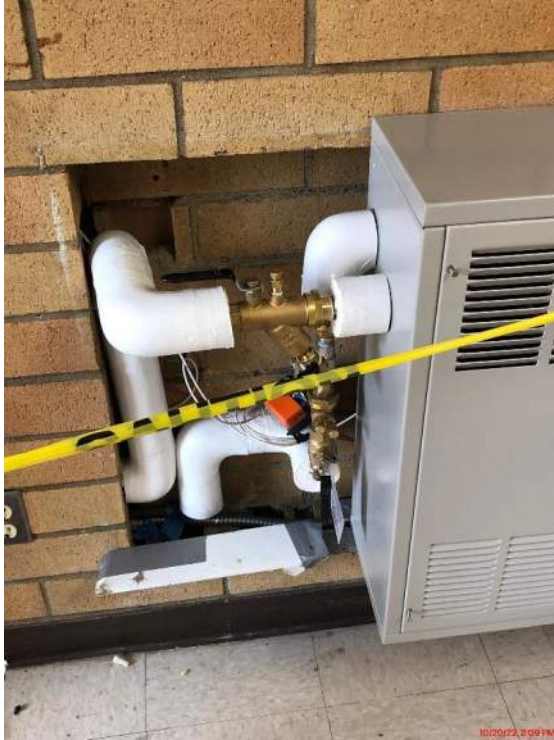
CMS – Cabinet Unit Heater Installation
