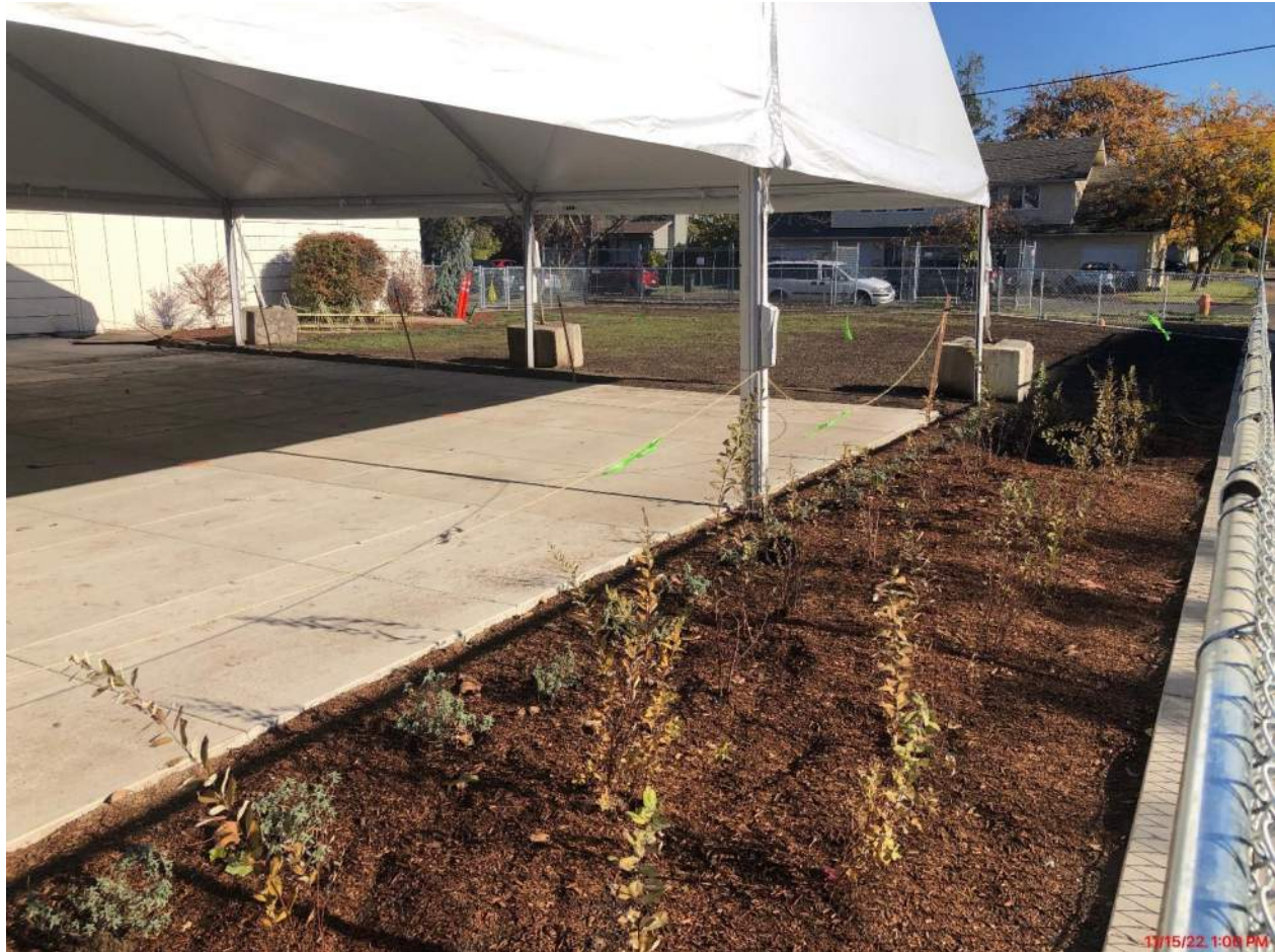
New Outdoor Patio landscaping & fencing
