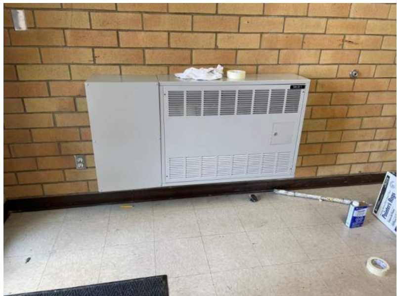
CMS – Cabinet Unit Heater Installation
