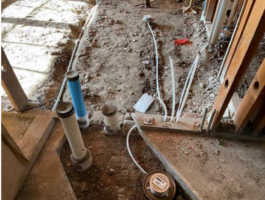
CHHS – Science plumbing underground progress
