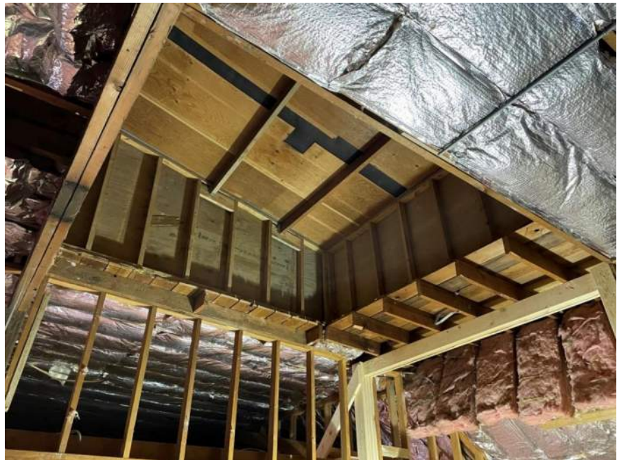
CHHS- temp roof framing to allow HVAC unit to be removed and reinstalled
