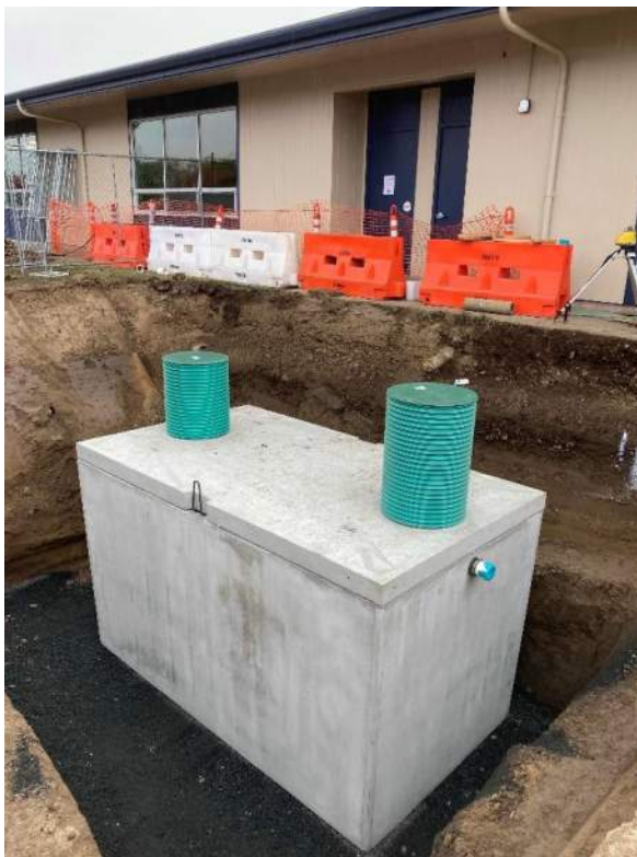
Installation of new septic tank
