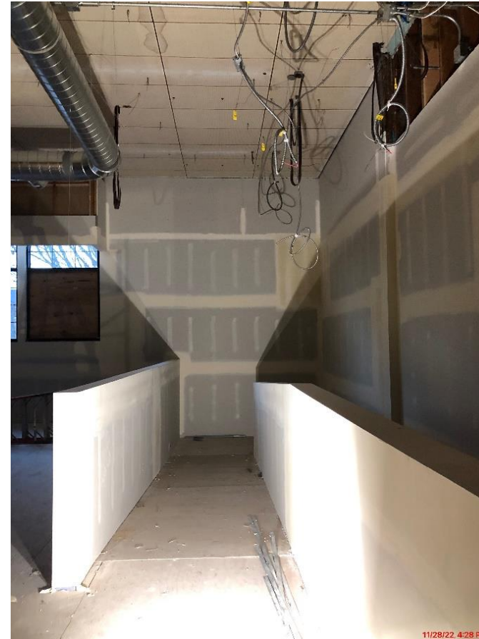
Library Ramp Wall Progress
