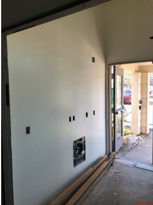
New Admin – finishes progress at entry
