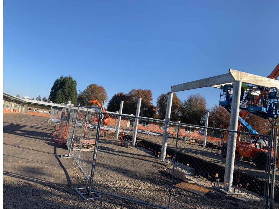
Covered Play Under Construction
