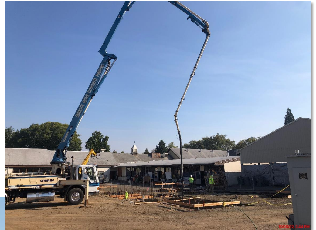
Pouring Footings for New Outdoor Classroom
