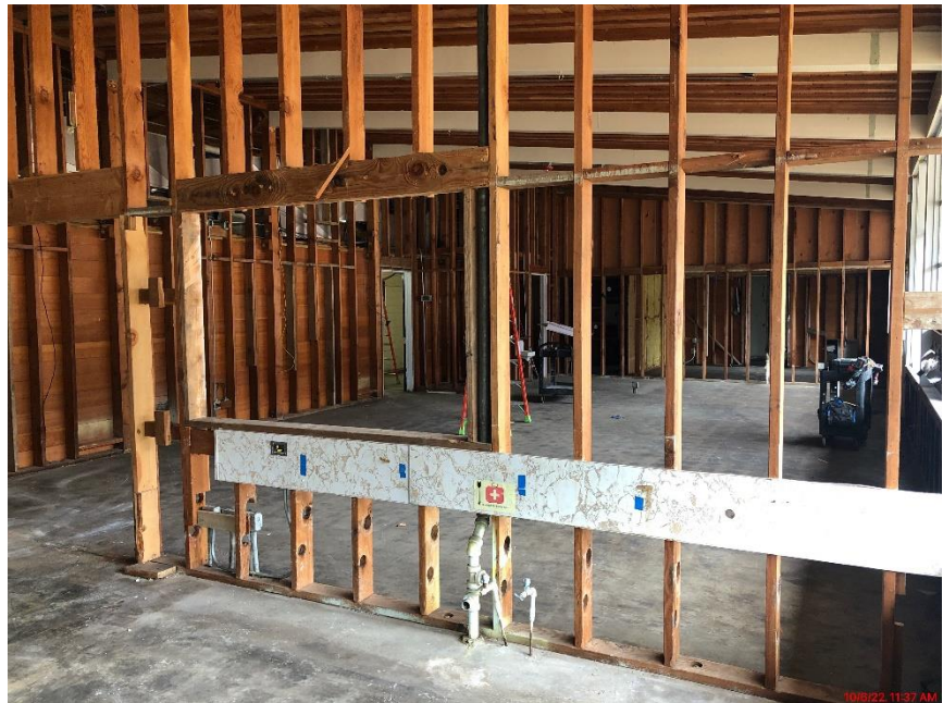
Area B Classroom Wall Demo
