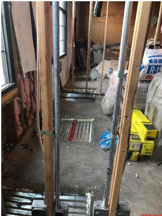
New Admin Tunnels Prepped for Slab Pourback
