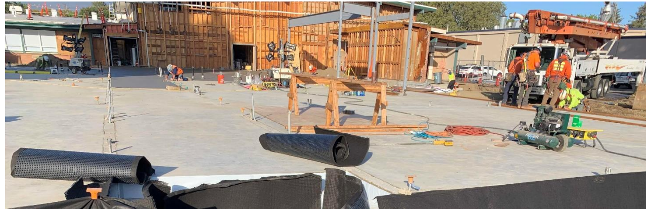
New Addition Slab
