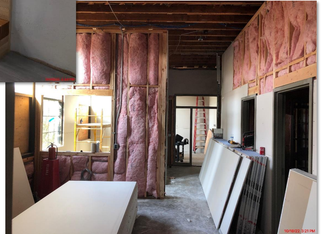
New Admin Space Progress
