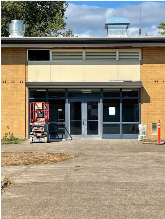
CMS – Louver Installation
