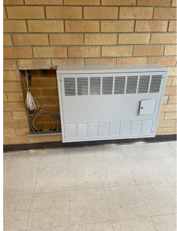
CMS – Cabinet Unit Heater Installation
