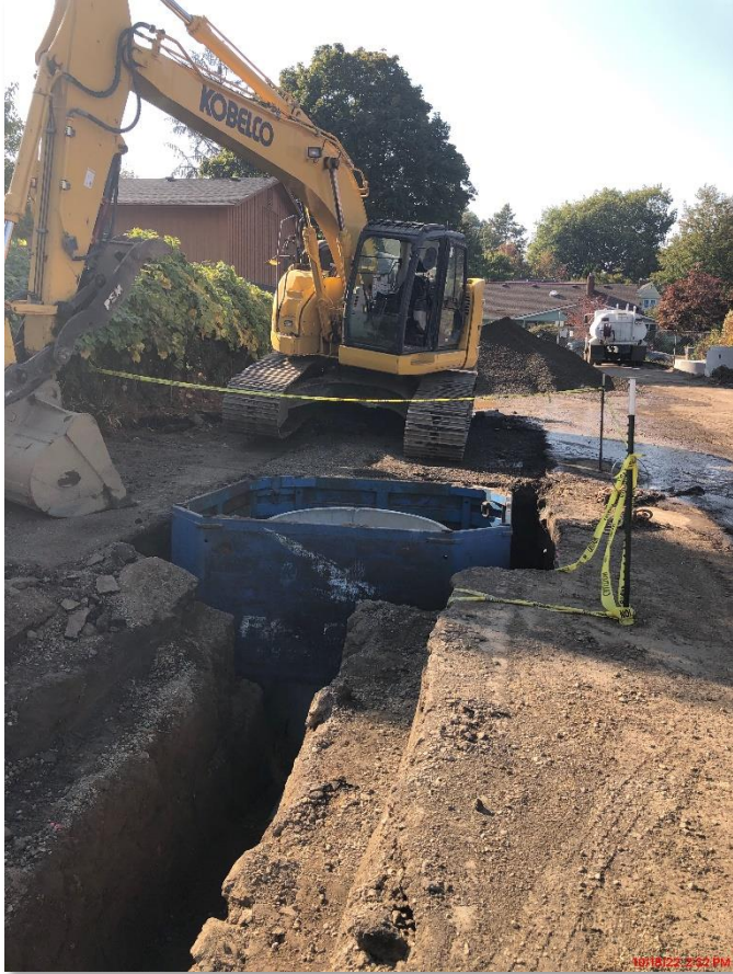
New On-Site Storm Manhole
