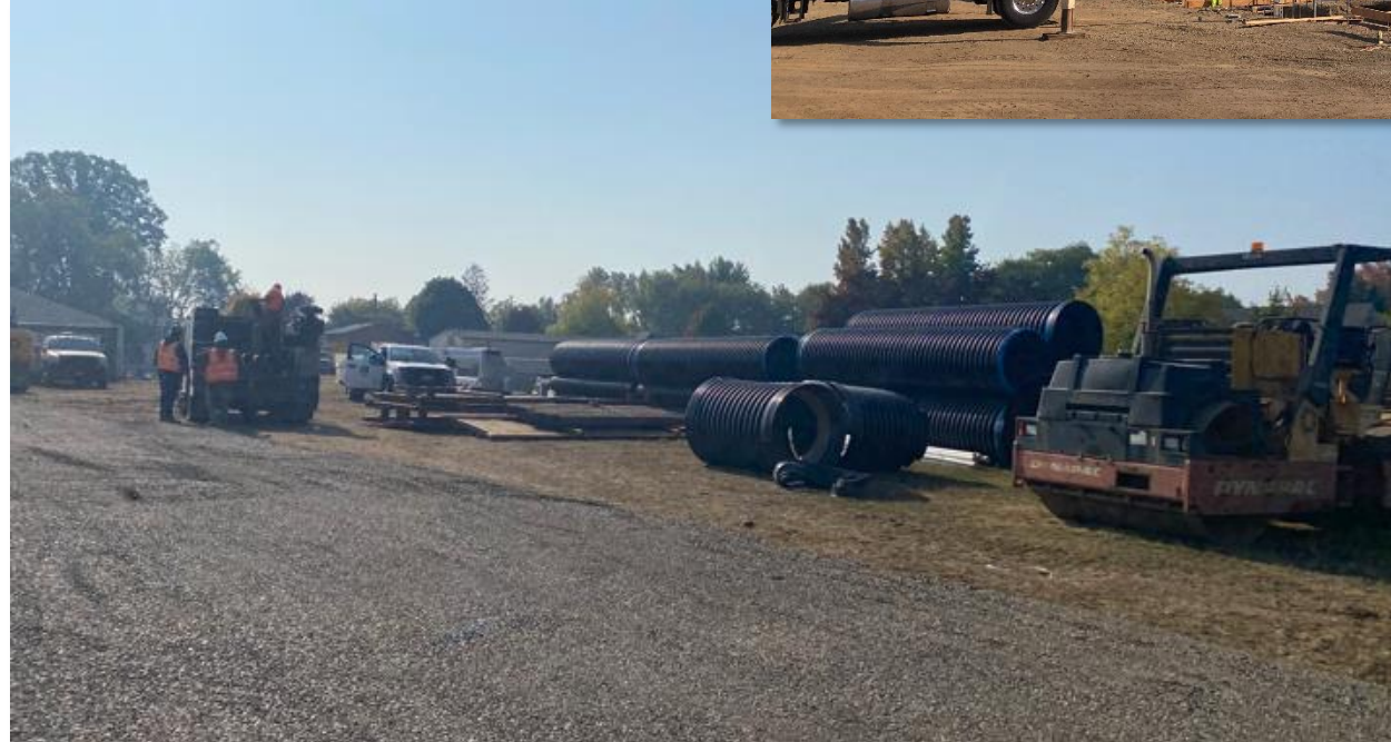
Storm Piping Staged
