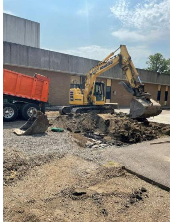
Cleanup between Bldg. A & B
