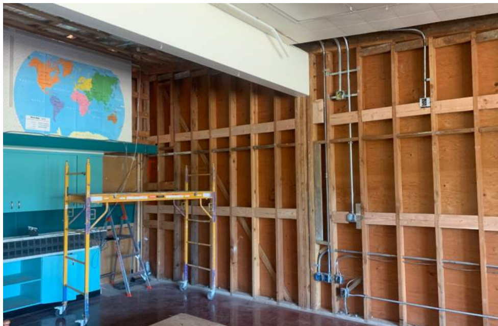
Classroom seismic blocking and technology rough-in
