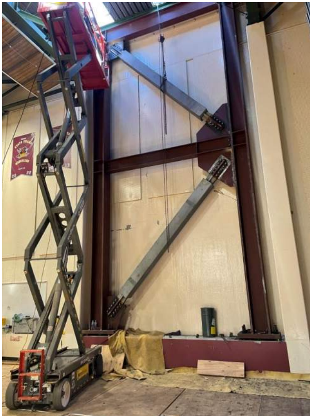
Bldg. A – Brace frame installed
