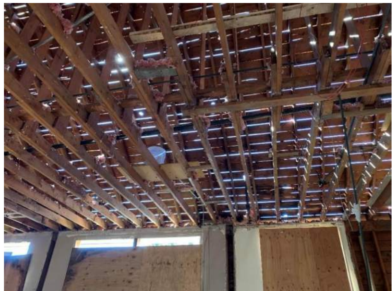
Office Ceiling demo progress
