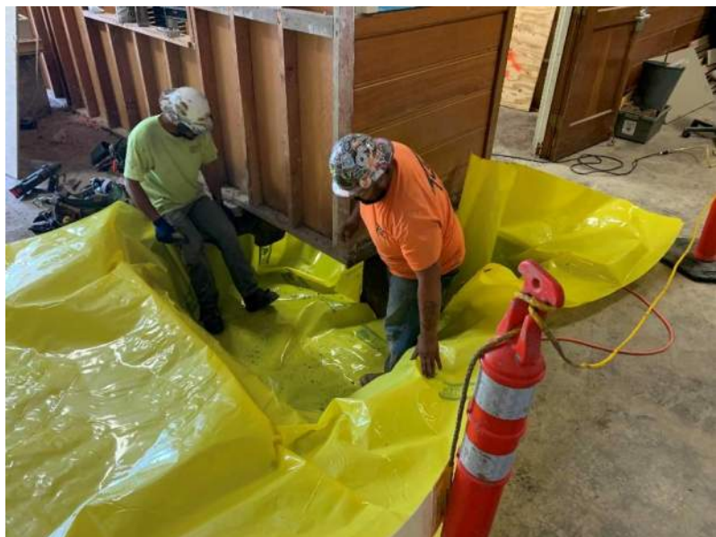
New interior footing work
