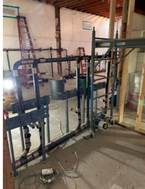
New plumbing rough-in
