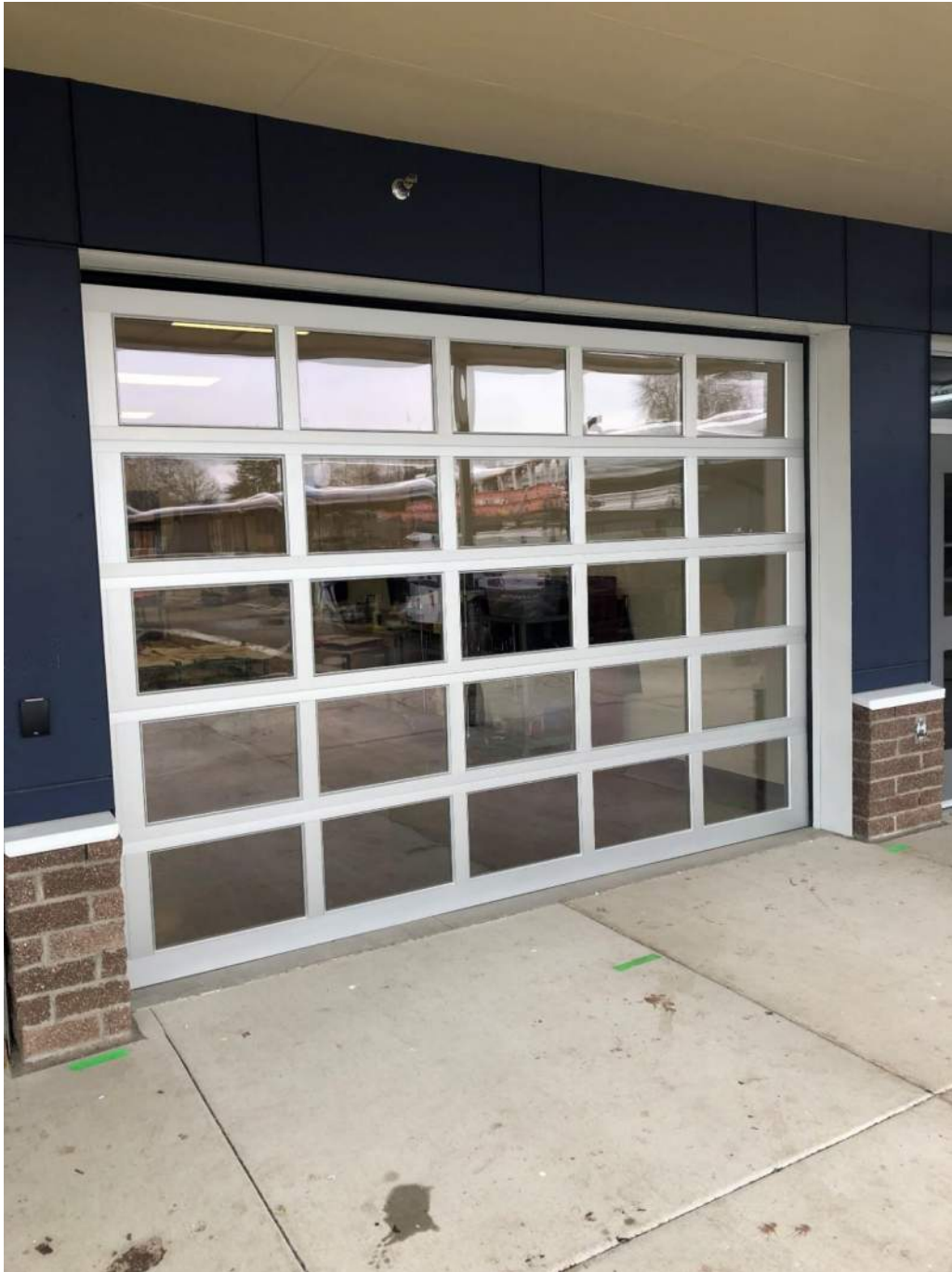
New outdoor classroom overhead door installed
