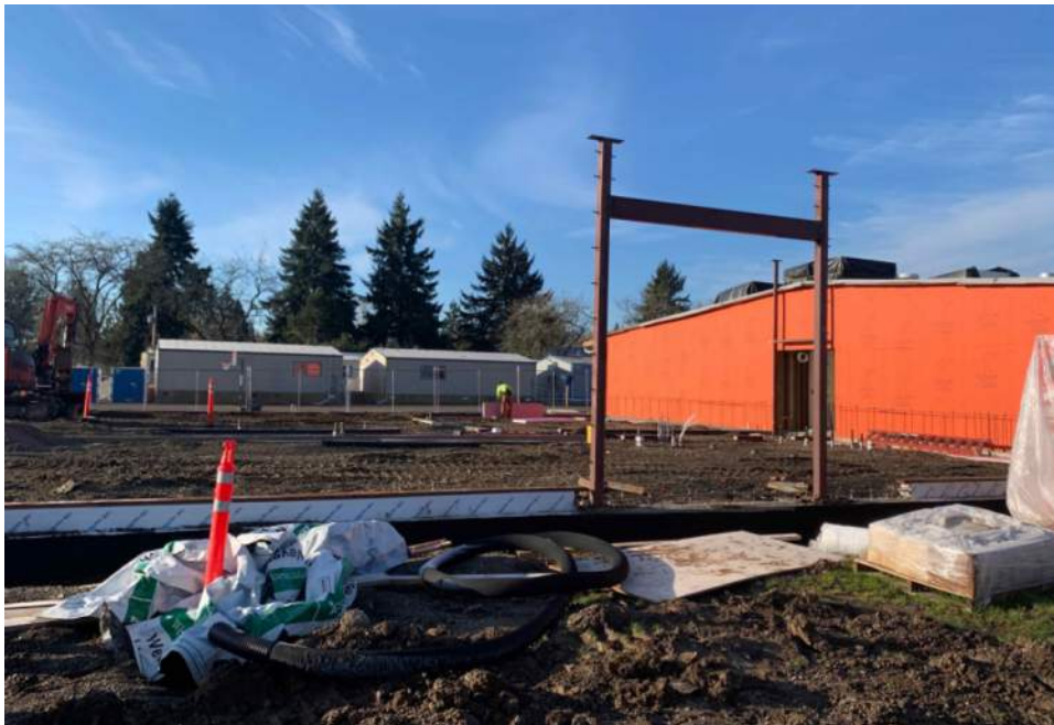
Slab Prep at Classroom Addition
