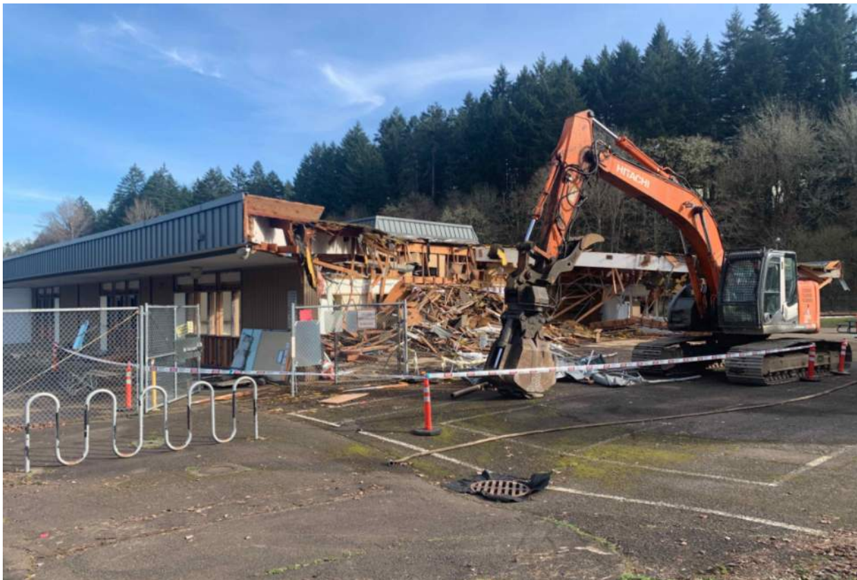
Demolition of Old Structure
