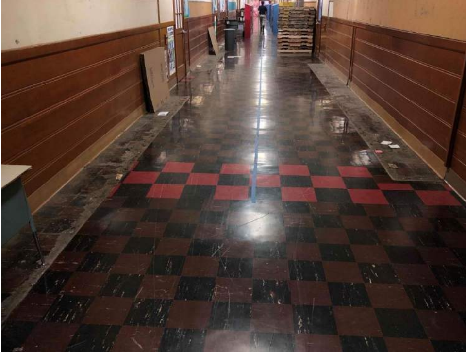
Franklin hallway after locker removal
