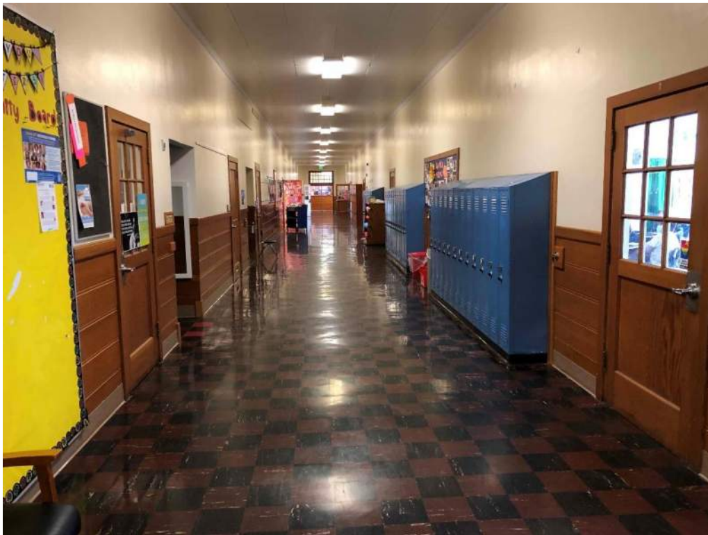
Franklin hallway before locker removal and flooring removal
