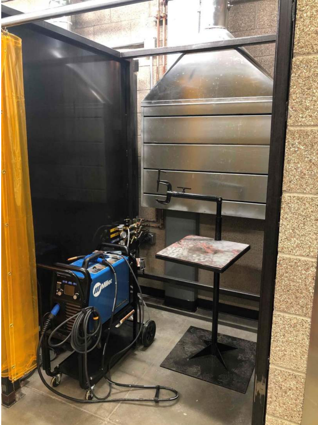
Completed Welding Booth
