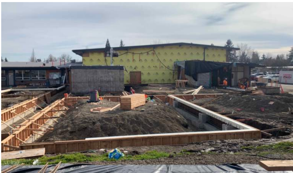
Footings for new classroom addition
