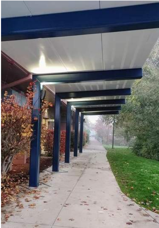
Covered walkway nearing completion
