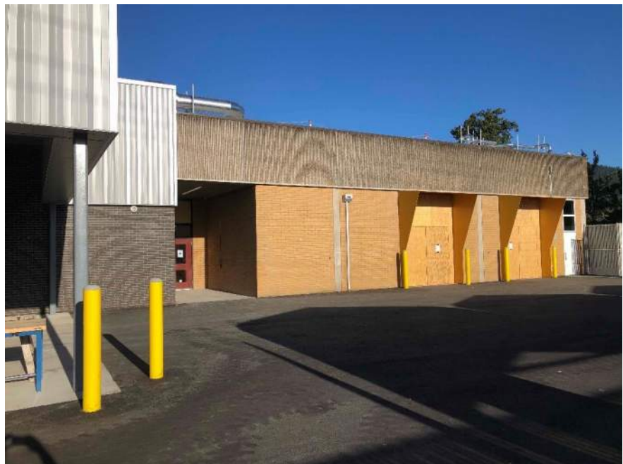
CVHS – Building F – Autos Yard
