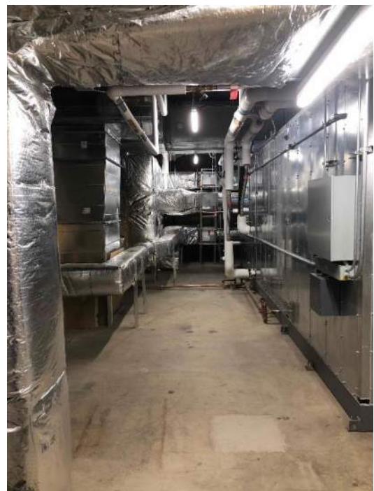
CVHS Building F – New mechanical mezzanine
