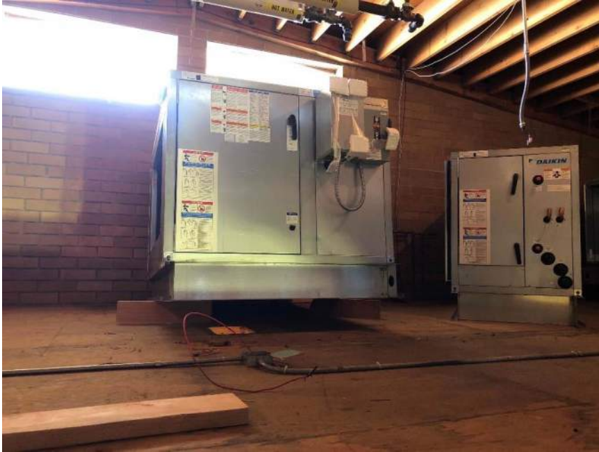
New HVAC installing at north mechanical mezzanine
