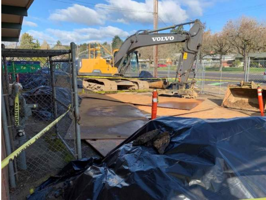
Oil Tank Removal
