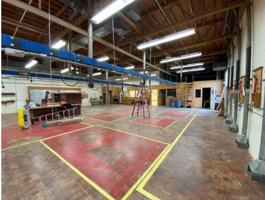
CHS woods ready for construction
