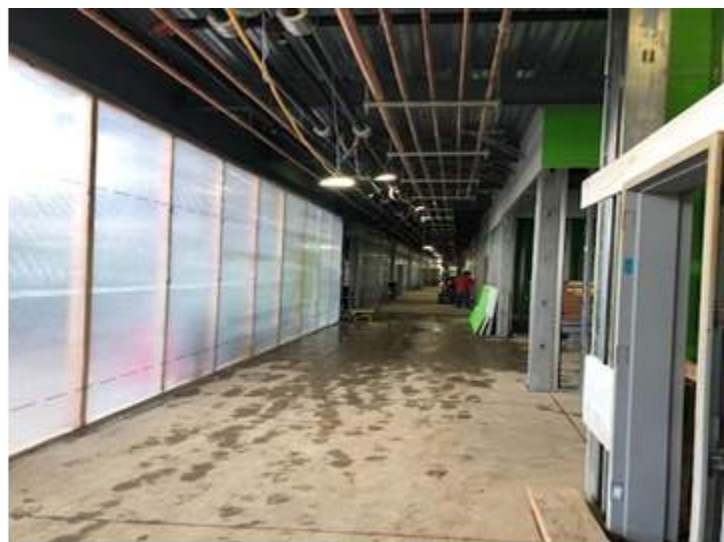
Interior framing and mechanical work underway
