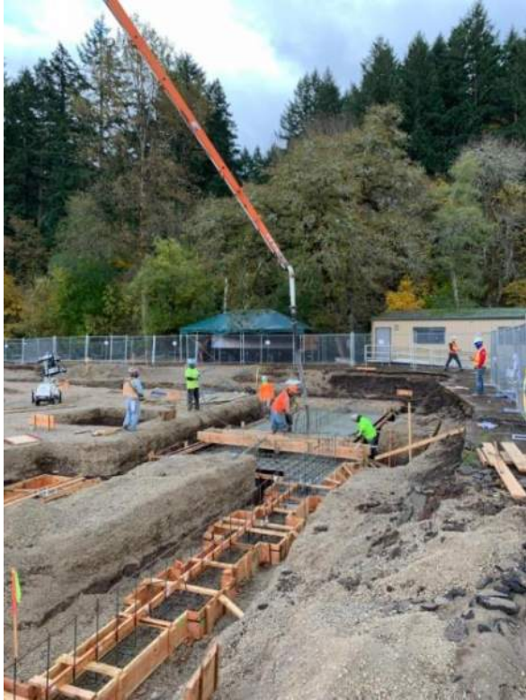
Pumping concrete into footings
