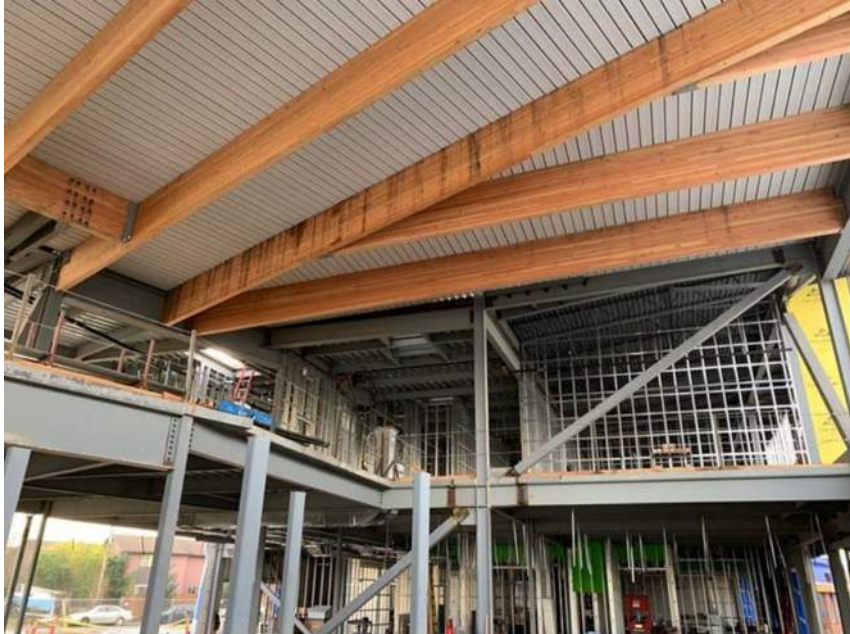
Commons area with exposed wood beams
