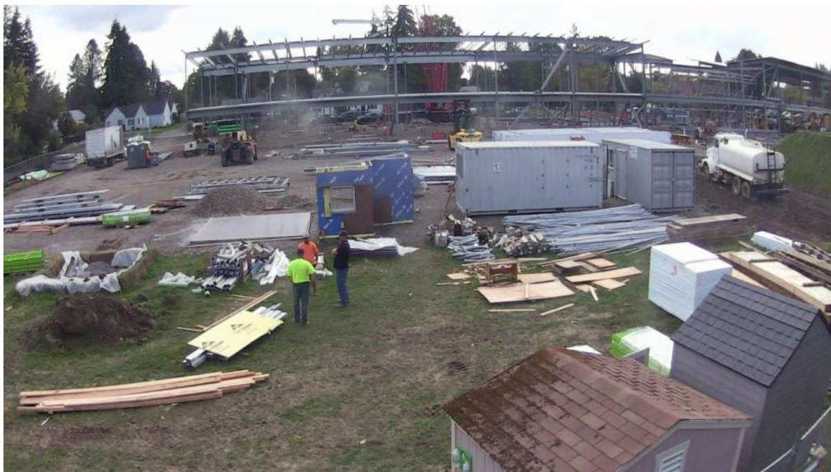
A webcam view of the LES site, dated 10/12/2020 showing the steel framing
