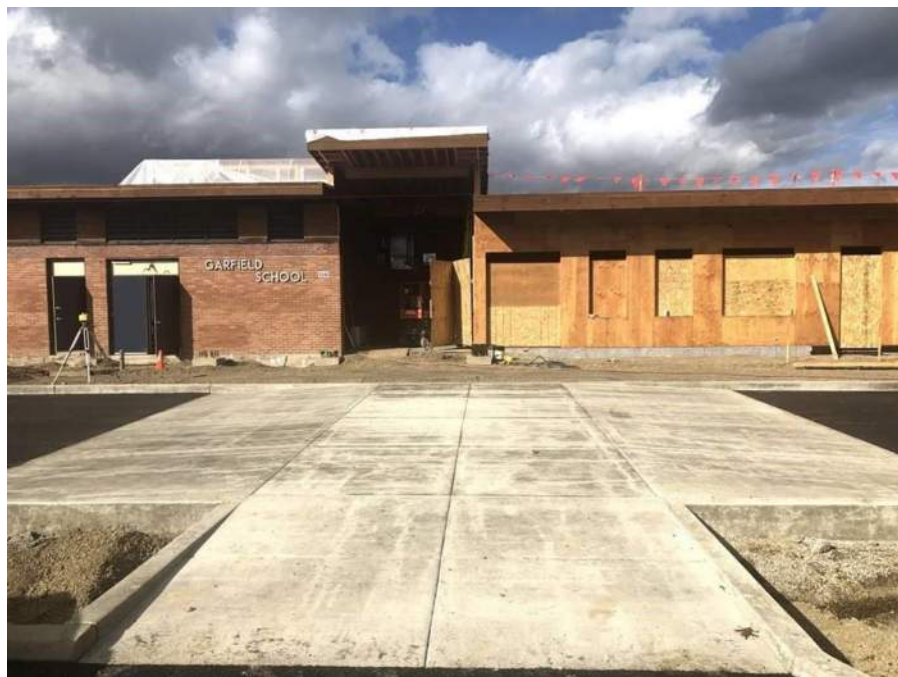
New front entry approach construction progress
