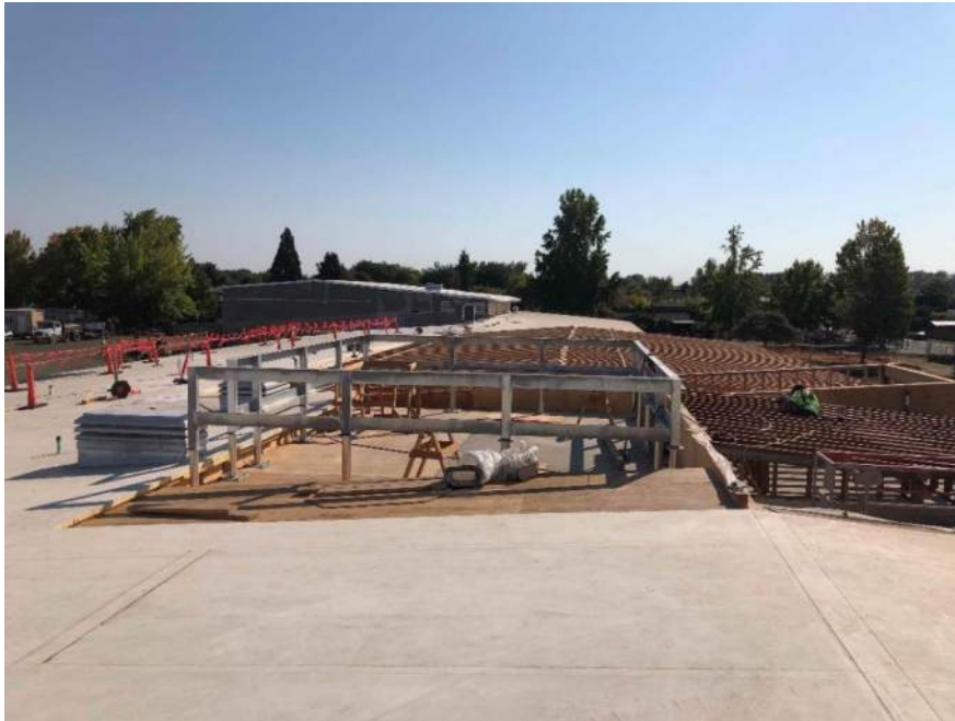
New office roof framing
