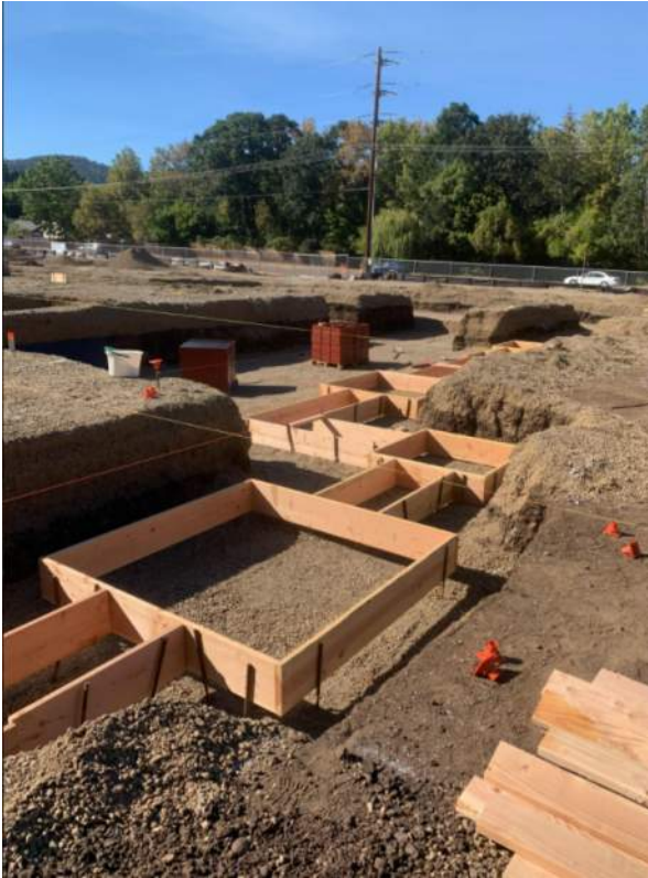
Footing formwork going in
