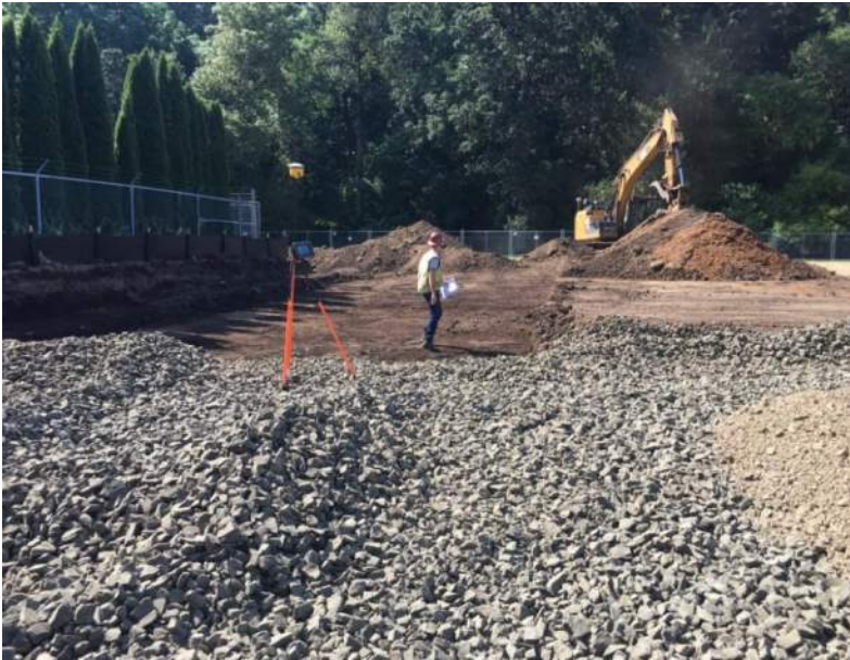
Removing soft soils and replacing with compacted gravel
