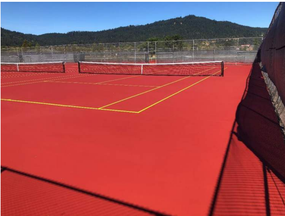
Tennis court resurface work
