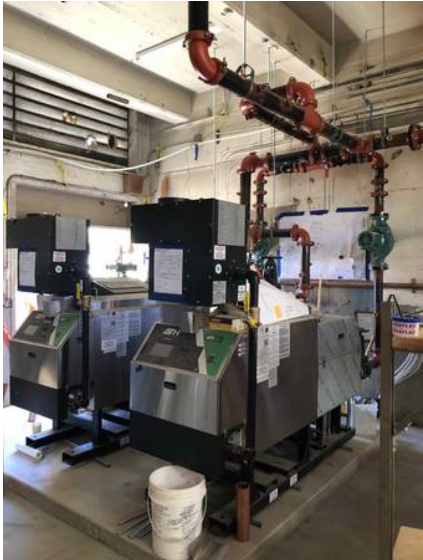
New boilers are installed and piping and electrical work are ongoing
