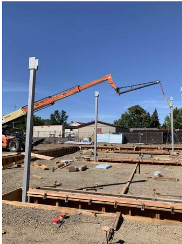
Steel erection at Clinic
