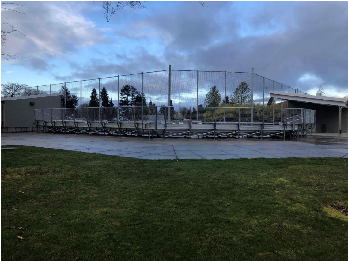
New bleachers installed at the softball field
