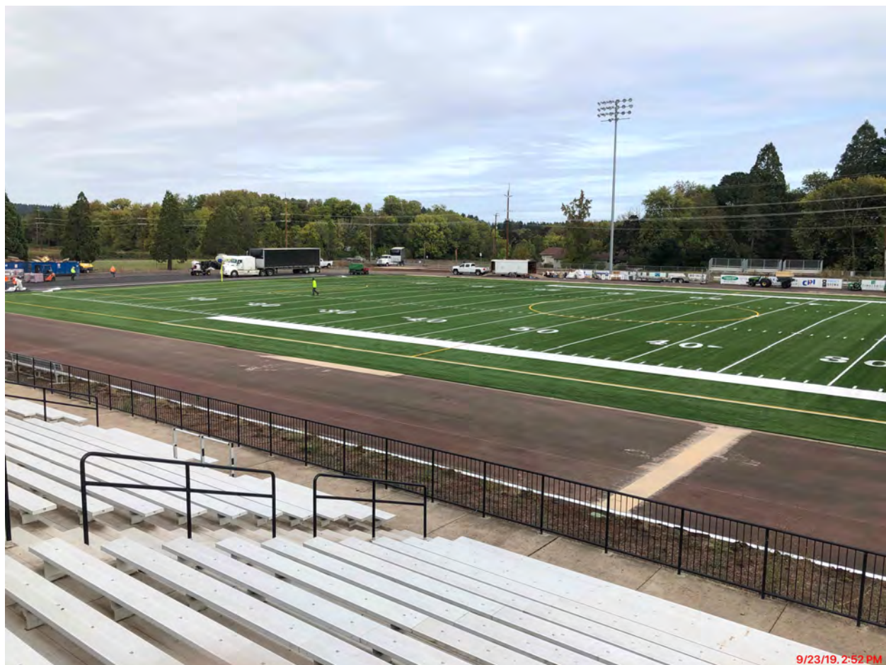
CVHS new turf field is complete
