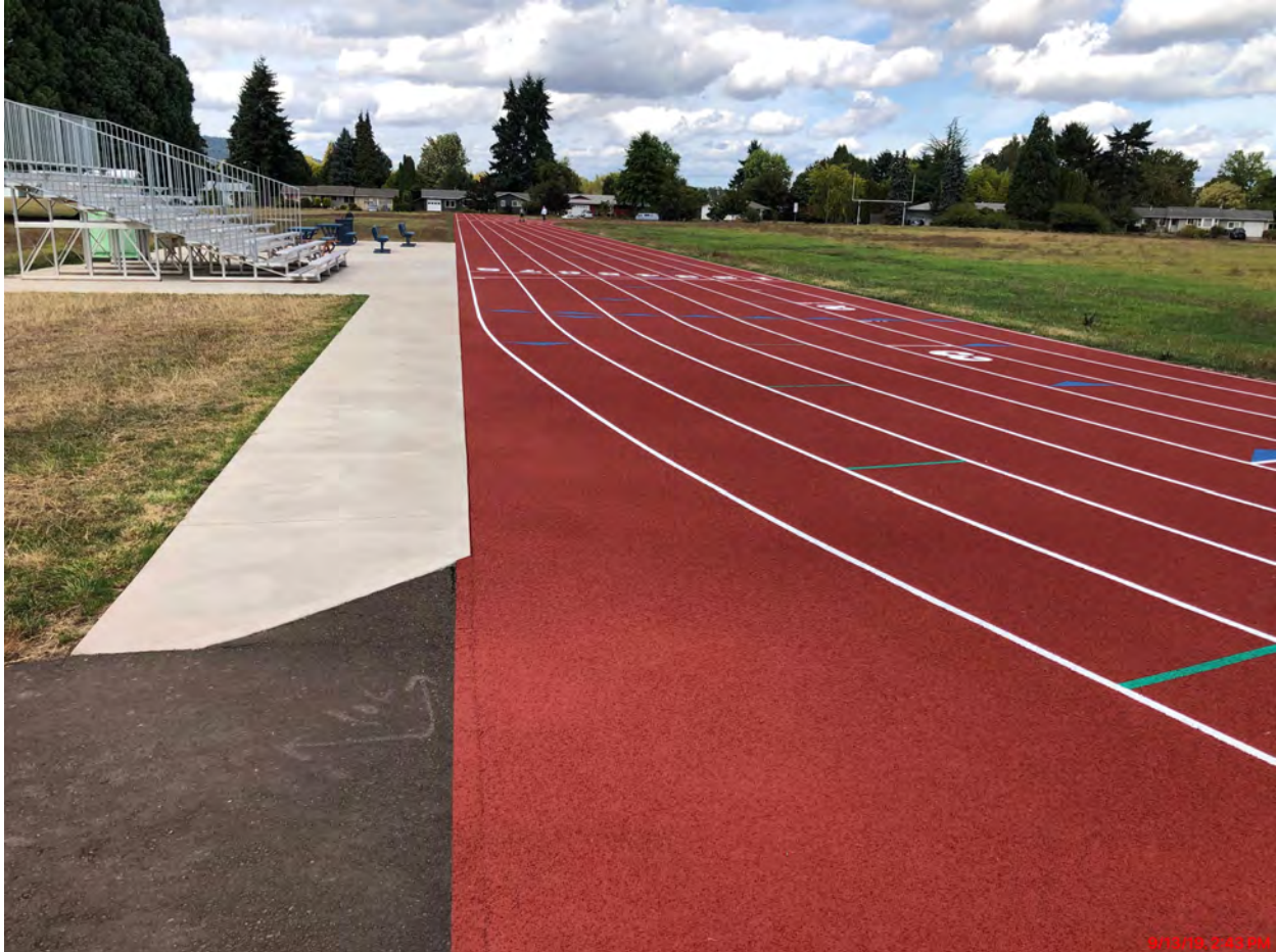
Track Resurfacing completed
