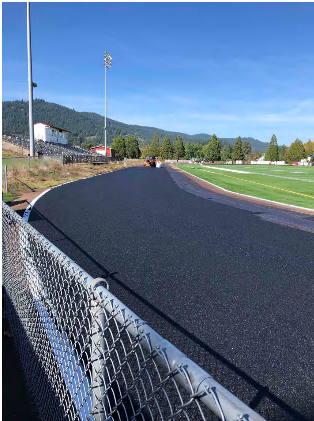
CVHS new track rubber surface going down
