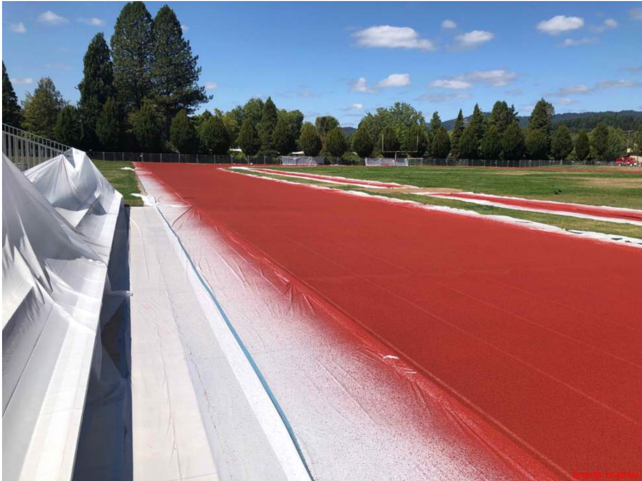
Track surface being applied
