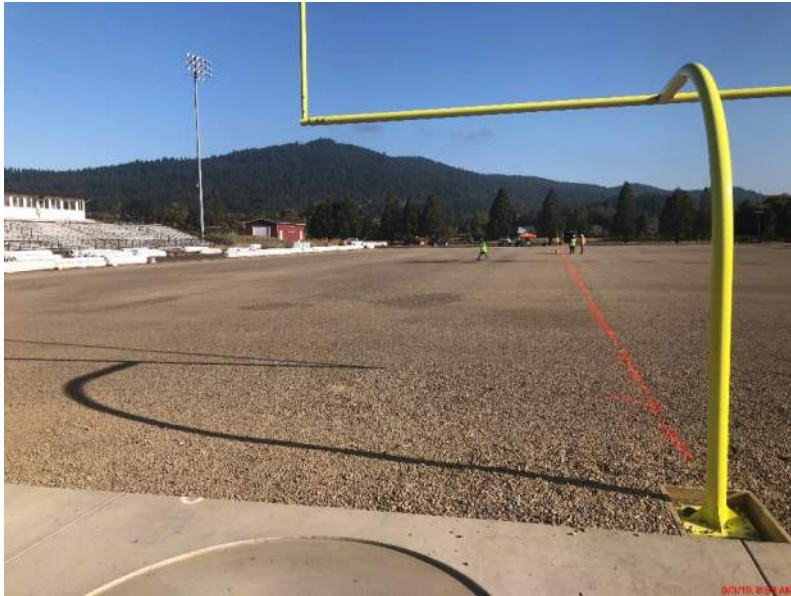
CVHS football field prepped for turf
