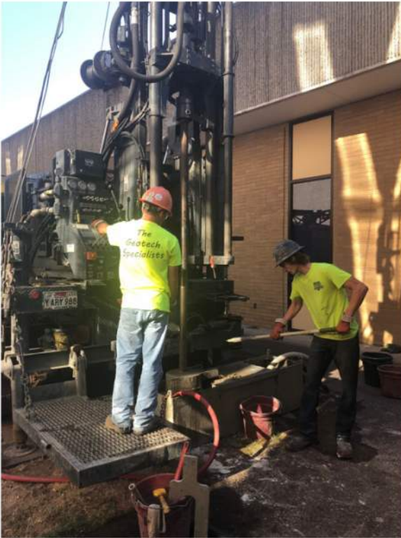
Additional Geotechnical boring to support future structural design
