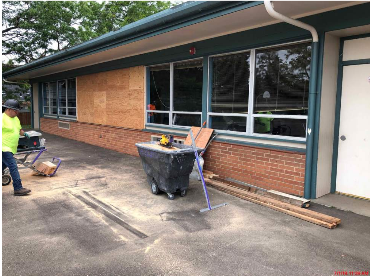
Infill at certain exterior windows to accommodate shear wall tie-in
