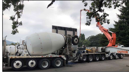
Pumping concrete curbs at track
