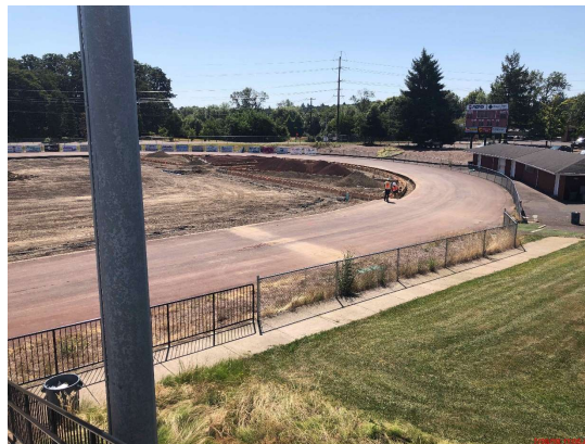
Track and athletic field work underway
