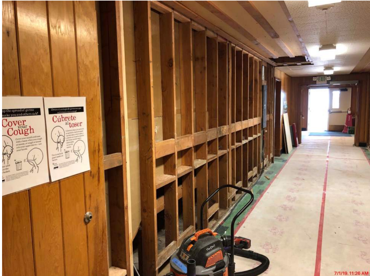
Demolition underway for Jefferson seismic project
