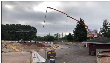
Pumping concrete curbs at track
