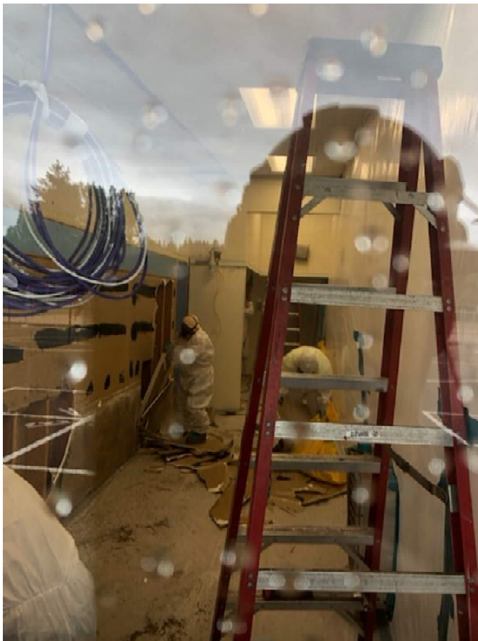
Abatement work in progress, photo through glass
