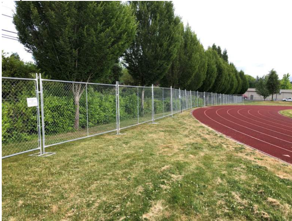
Tree Protection installed
