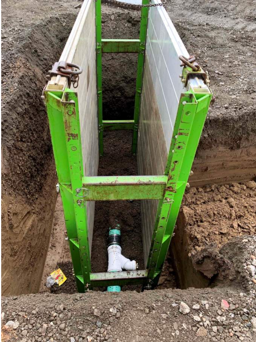
Contractor utilizing appropriate safety devices for deep excavations
