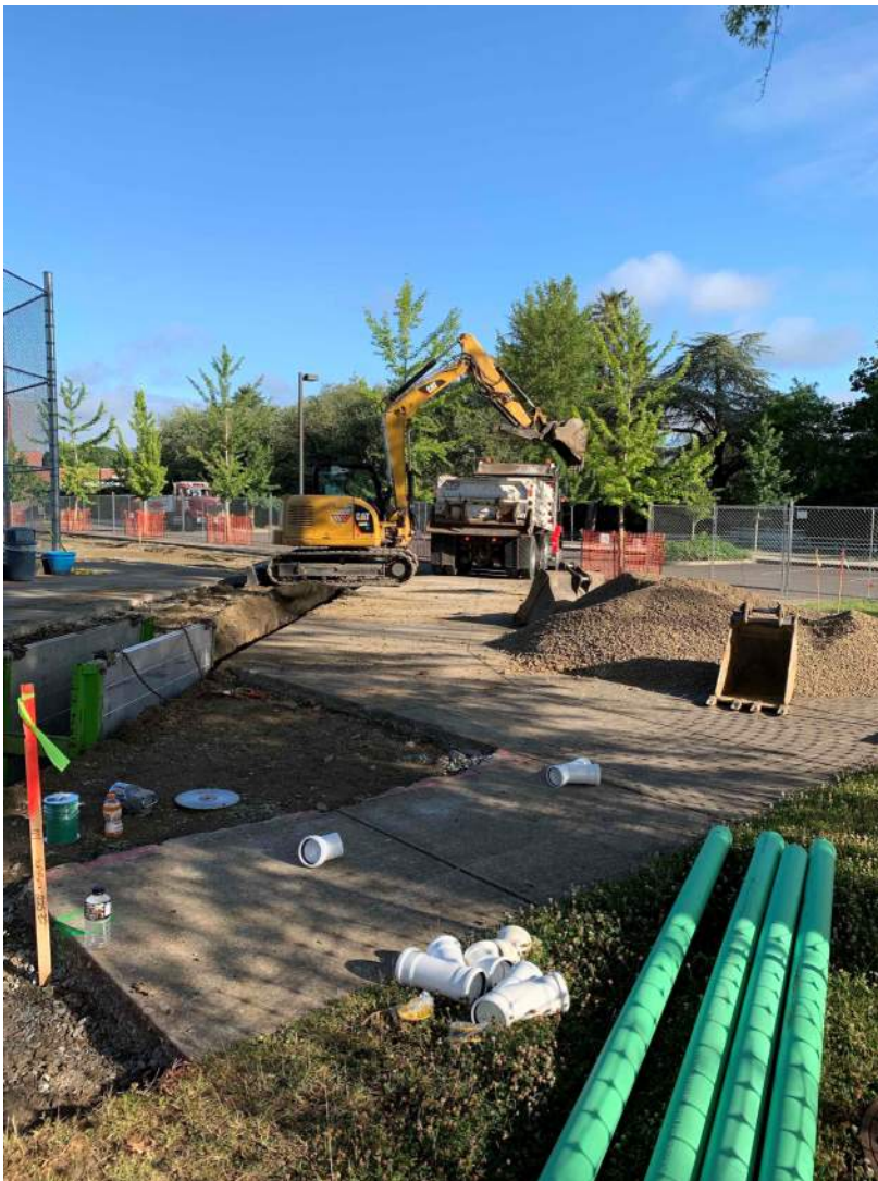
Excavation begins at the CHS Softball field
