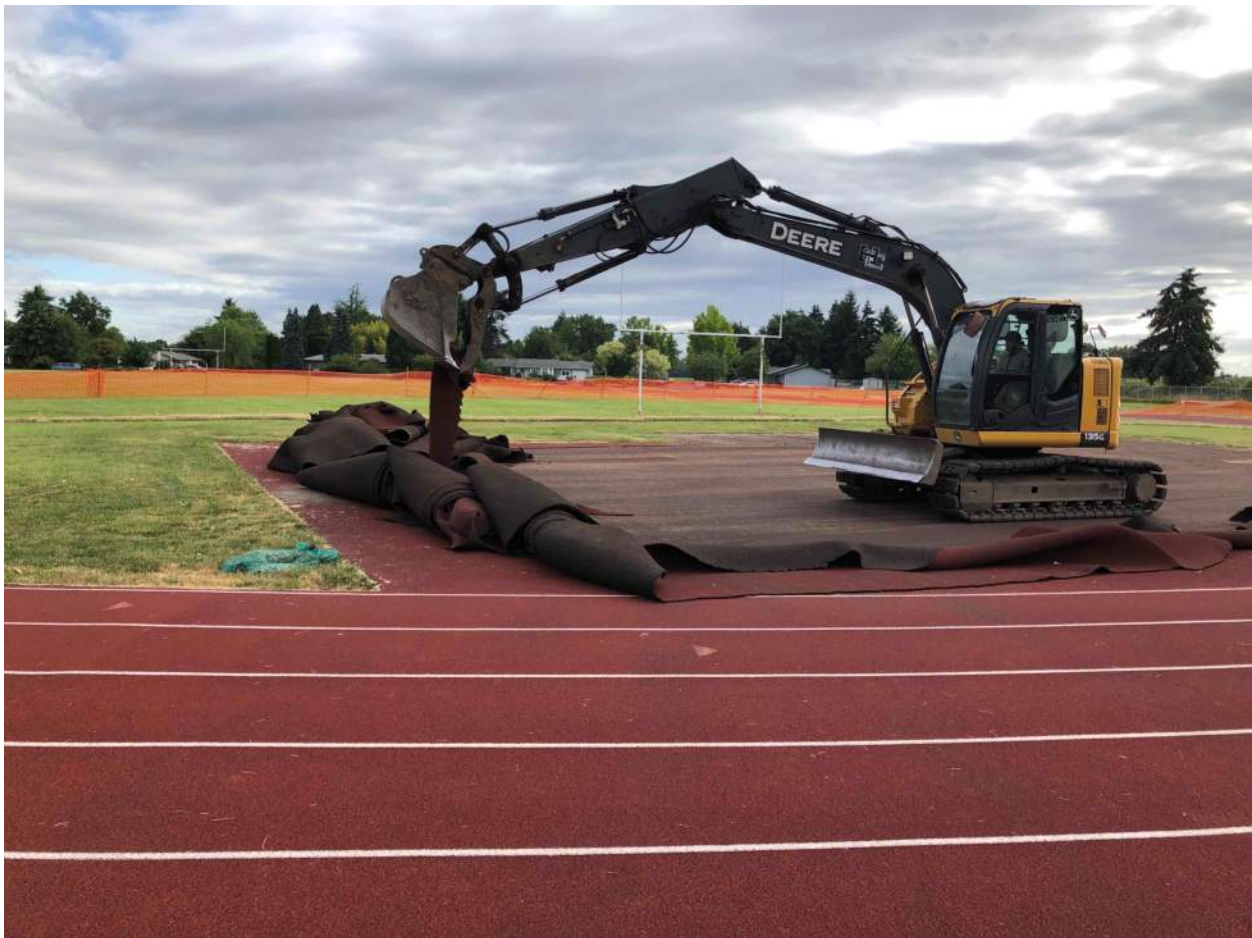
Track Demolition begins
