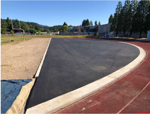
D-Zone asphalt work
