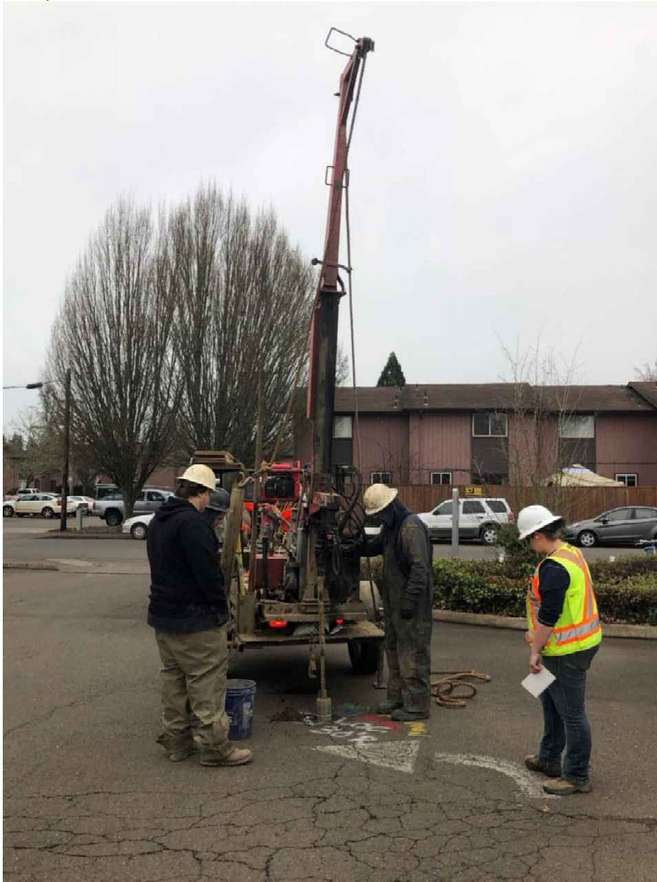
Workers from Foundation Engineering and Western States Drilling perform drilling for the geotechnical survey
