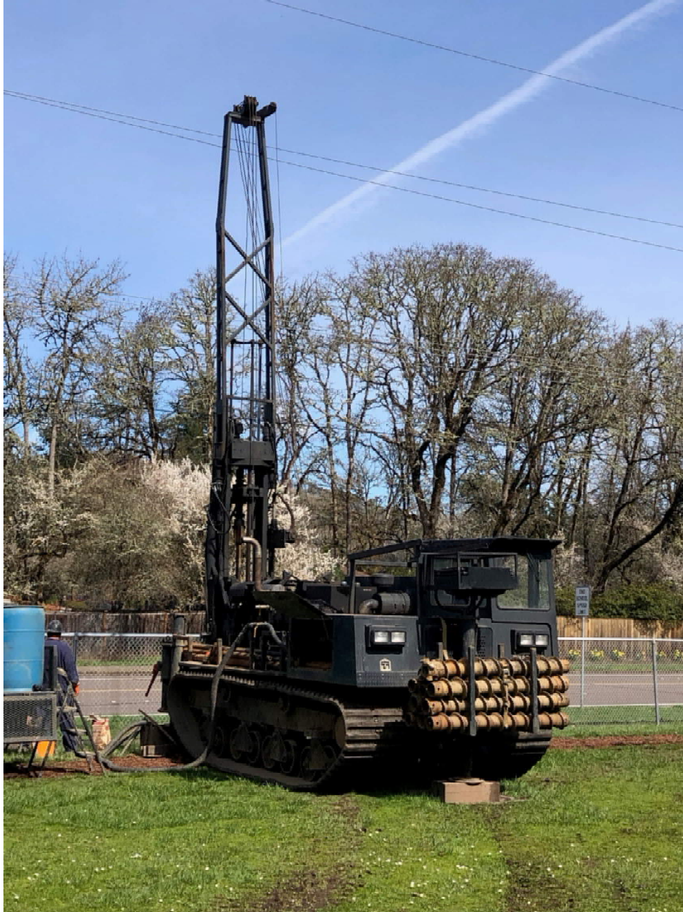
Drilling for geotechnical survey at Hoover Elementary
