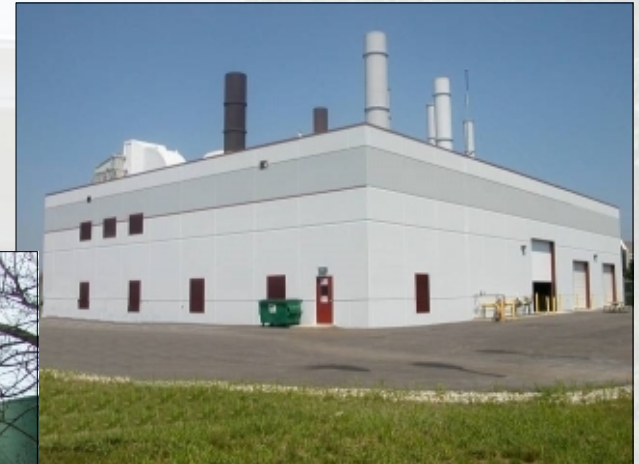
North Chicago Energy Center Chicago, Illinois Over $10 Million in Operations and Maintenance Savings
