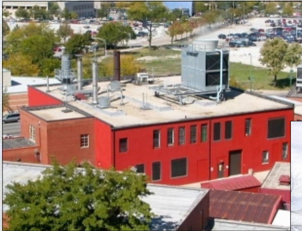
West Side Chicago Energy Center Chicago, Illinois Energy and Operational Savings Over $30 Million
