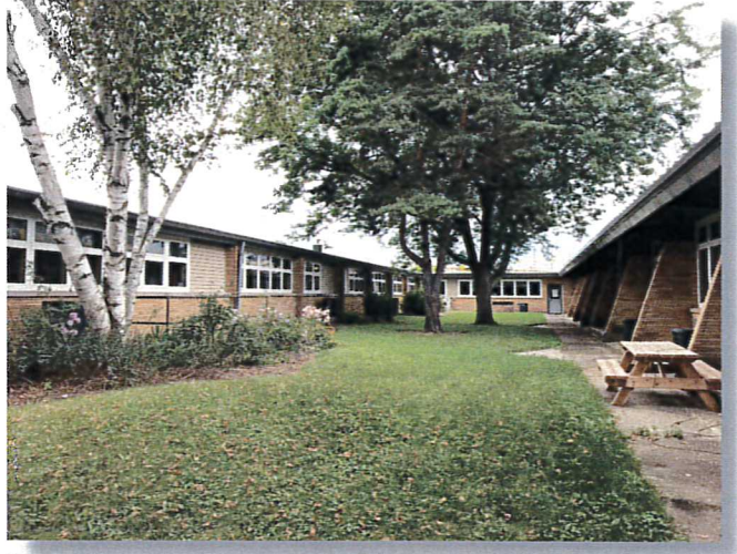
Courtyard View of New Glarus Elementary School
