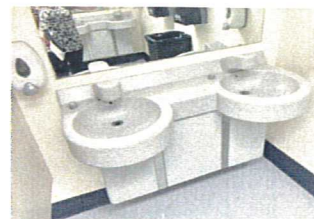
Main Toilet Room Lavatories
