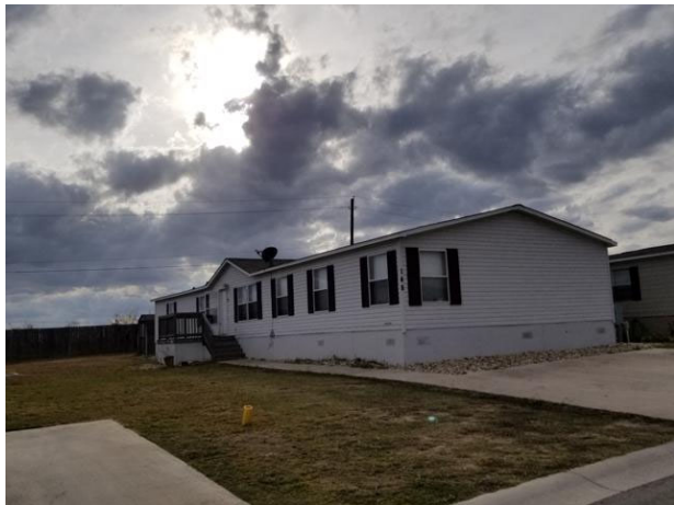
View of adjacent trailer home (Borders the easement to the west)
