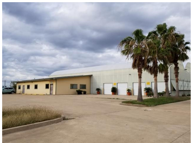
Vickery Wholesale Greenhouse along Daffan Lane (Across from the easement)
