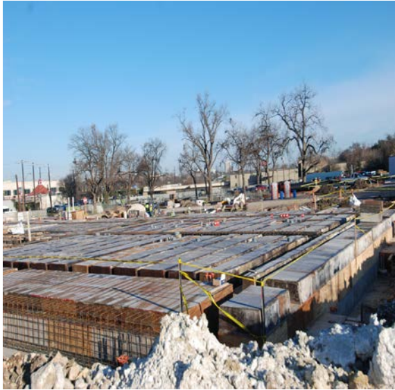
Building B, C
