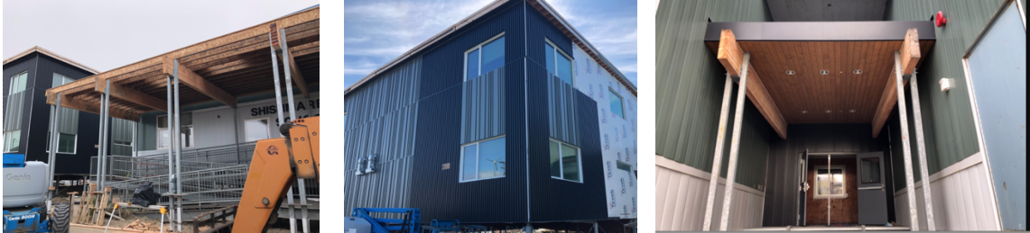
916 917 Exterior work taking place on The Shishmaref School this summer
