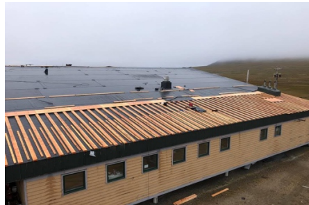
New roofing being installed
