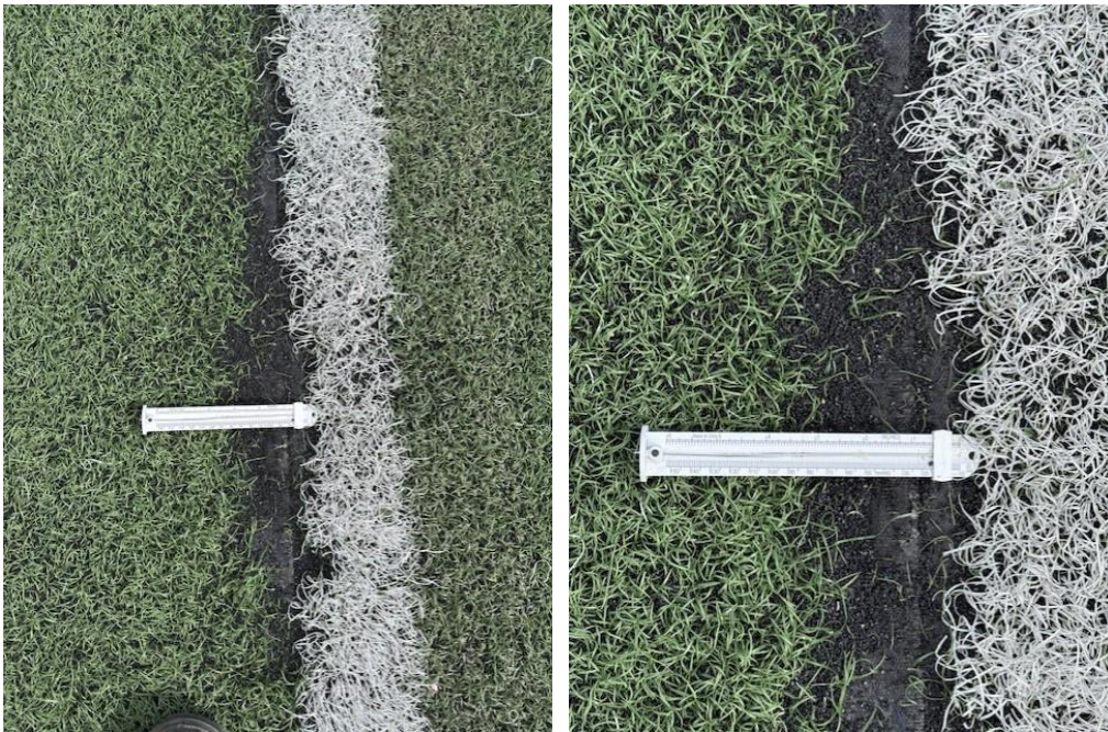
Seam separation on the white lines of the East side. (4 inch wide and some 30-60ft long)
