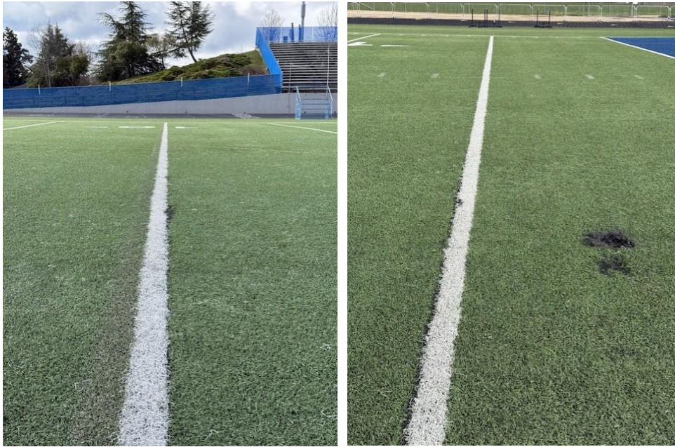
Seam separation on the white lines of the East side. (4 inch wide and some 30-60ft long)
