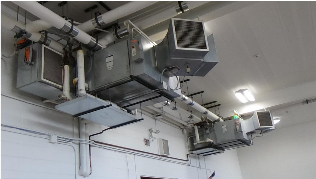
Euclid School Multi-Purpose Room
