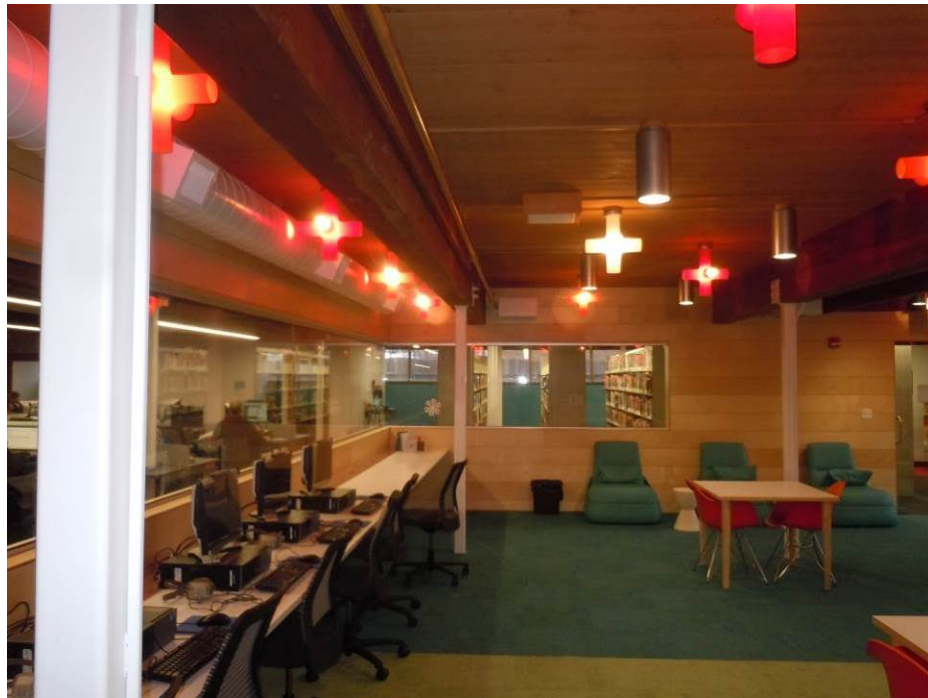
24. Southeast, lower level Teen Center with new lighting, air distribution and data outlets
