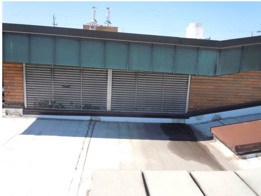
21. East Roof looking South, with AHU-1 exhaust louver, Chimneys
