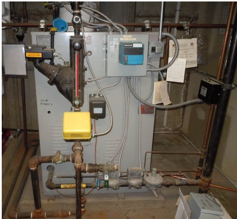
8. Humidifier Boiler, 1997
