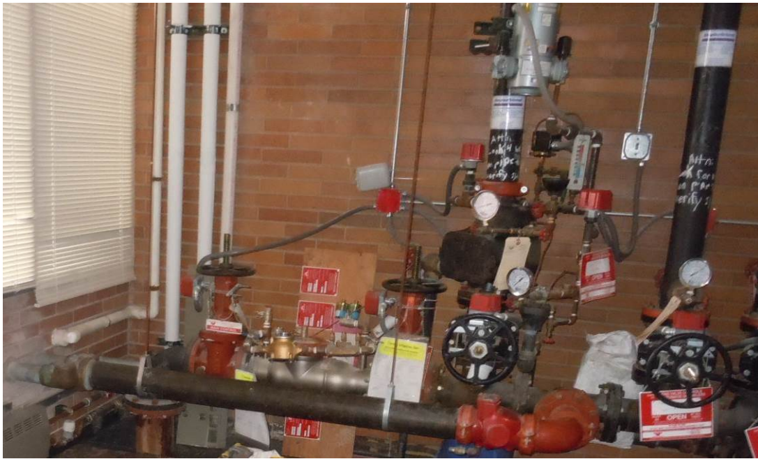
32. Fire Protection Water Service, adjacent to main meeting room
