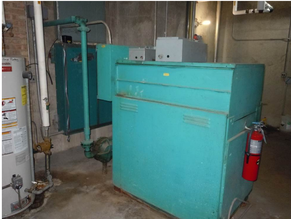
30. Original Elevator Equipment, Abandoned in NE basement
