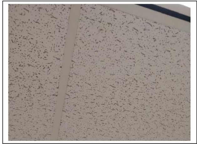
Photo # 6 2'x4' Ceiling Tile Small Pin Holes with Gouges Classrooms 126, 132, 133, 134, 135, 136, 137, 138, 139, 140, 141, 142, 143, & 144 Negative for Asbestos
