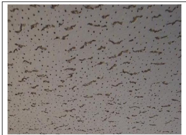
Photo # 4 2'x4' Ceiling Tile – Dot and Gouge Pattern Classrooms 103, 104, 105, 112, 113, 114, 115, Learning Center, 118, 119, 120, 121, 122, Adjacent Corridors, 127, 128, 129, 130, 131, & 131A - Negative for Asbestos
