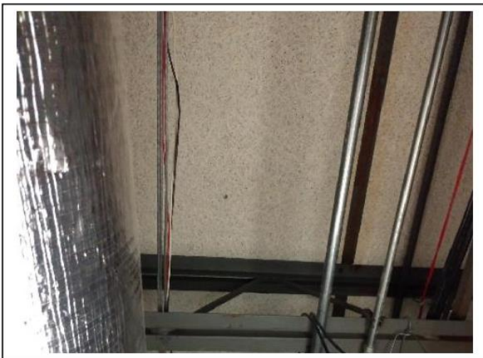
Photo # 7 Tectum Ceiling Panels Negative for Asbestos
