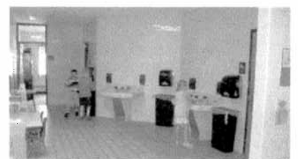
Wildwood East Wing Restrooms
