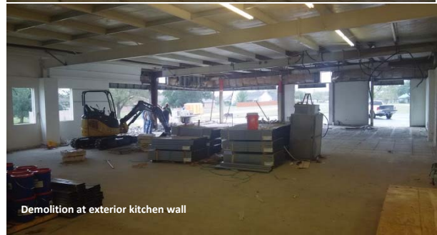
Demolition at exterior kitchen wall
