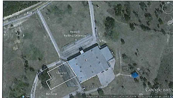
Shady Grove Elementary School Campus Improvement
