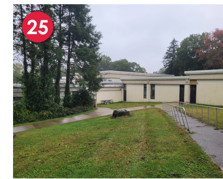
Biofiltration Swale Revegetate Slope Drainage Area 5
