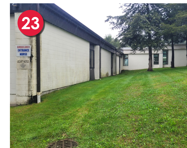
Rain Garden Drainage Area 5
