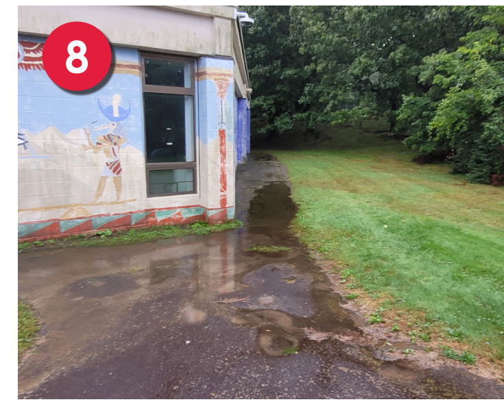
Rain Garden Drainage Area 1
