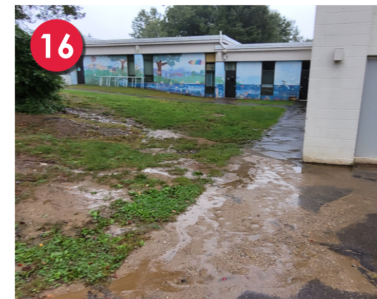
Rain Garden Drainage Area 1
