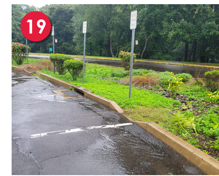
Remove Pavement New Pervious Pavement Drainage Area 2
