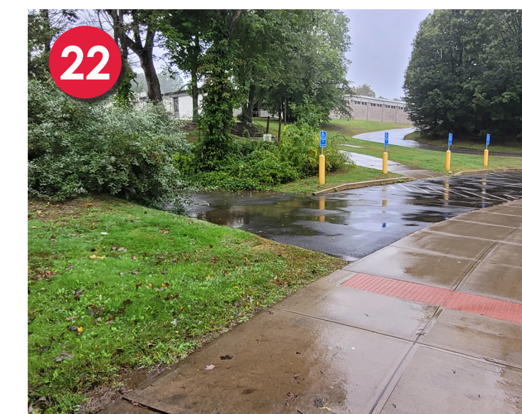
Pervious Pavement Drainage Area 4
