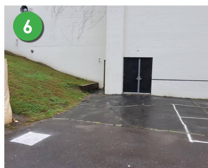
6 Remove Invasives Revegetate Slope Drainage Area 1
