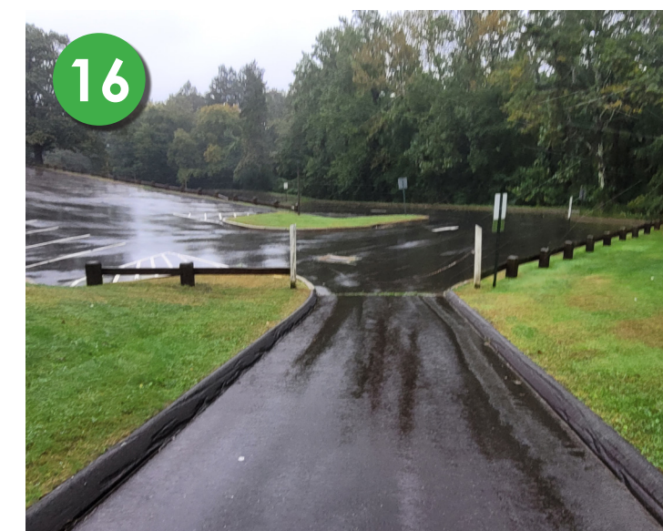
16 Woodland Buffer Remove Invasives Drainage Area 6
