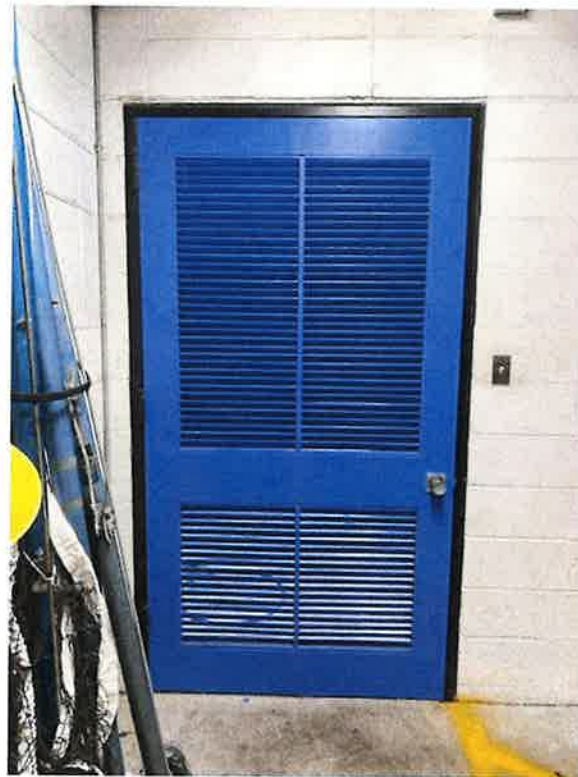
Louvered door in Gym storage room
