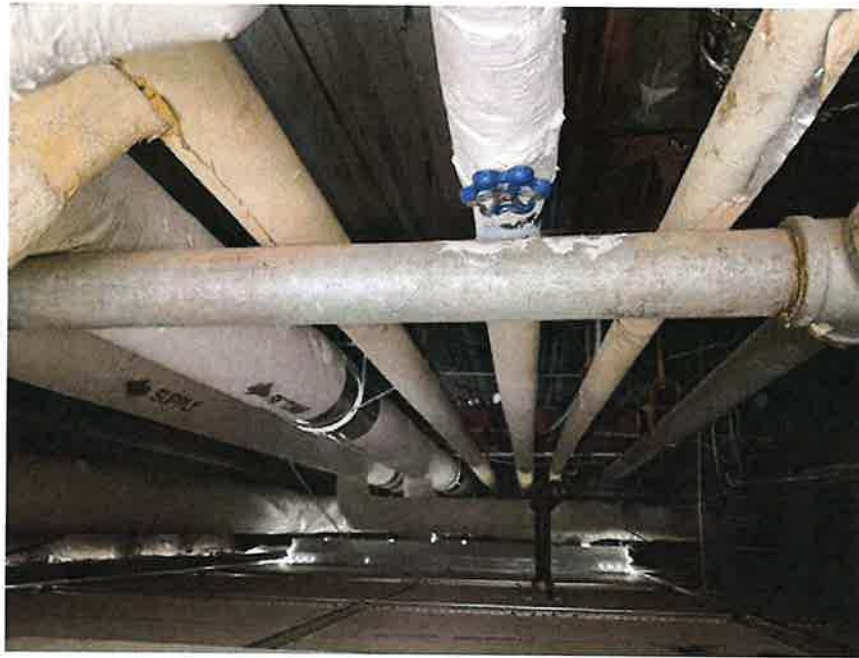
Ceiling space in Corridor area
