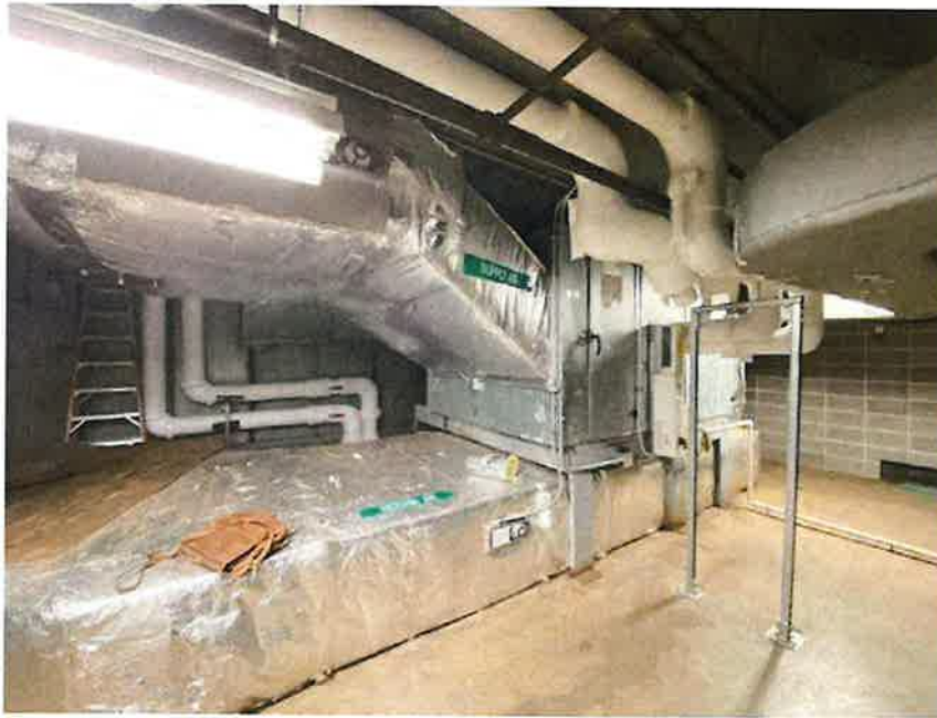
Existing Cafeteria unit Where heat pipe will be installed
