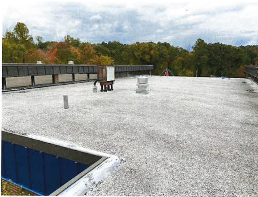
Lower roof where new DOA units will be placed
