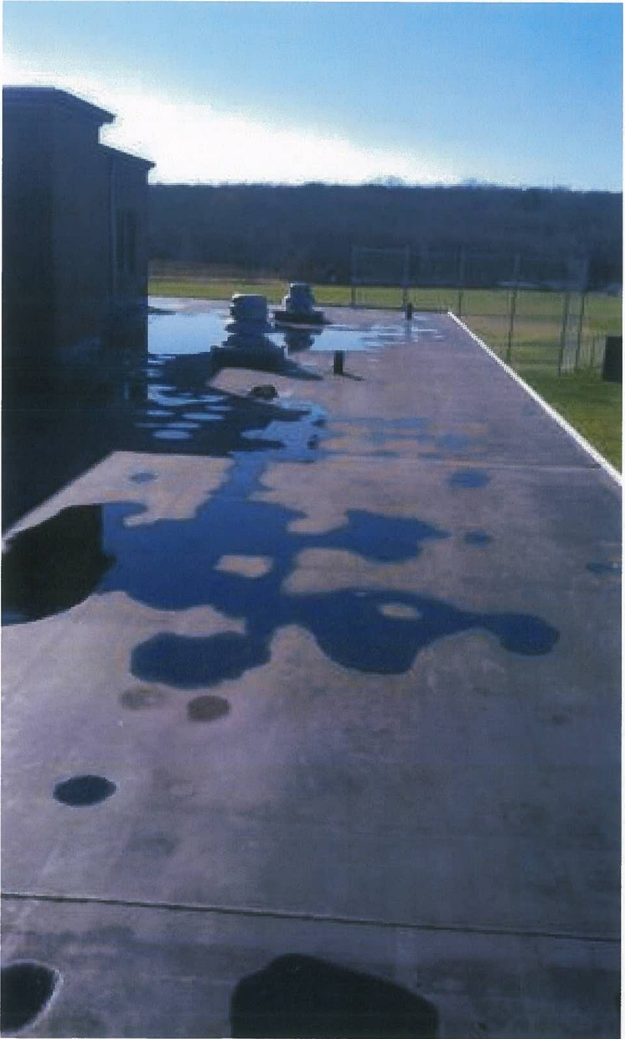
Boys' Locker Room
