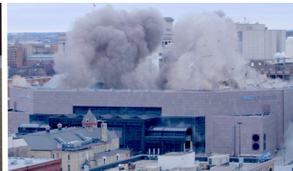
BMO HARRIS BRADLEY CENTER DEMOLITION
