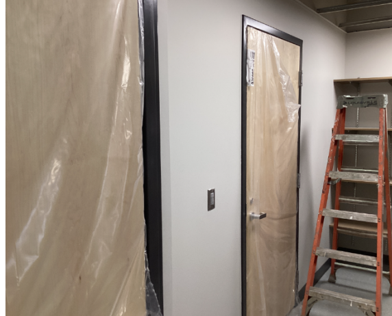
New Door Installation
