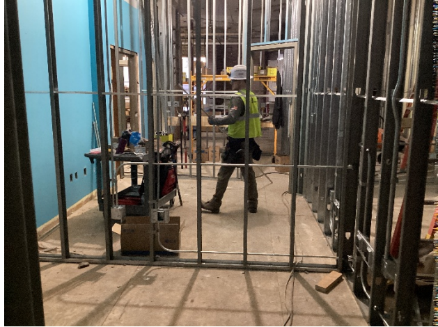
1st Floor MEP Rough-In
