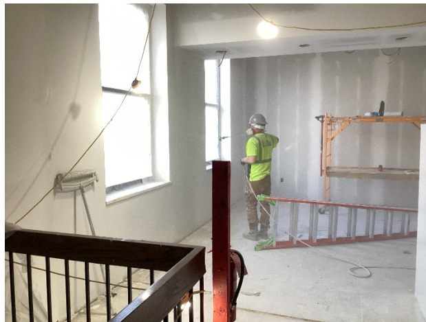
2nd Floor Painting Continues
