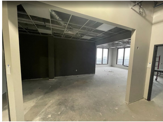
2 nd Floor Ceiling Grid
