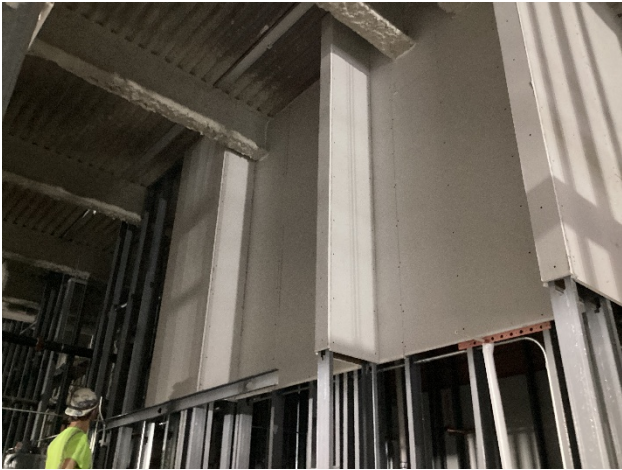
1st Floor Drywall Installation
