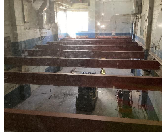
1 st Floor Structural Steel
