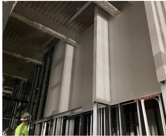
1 st Floor Drywall
