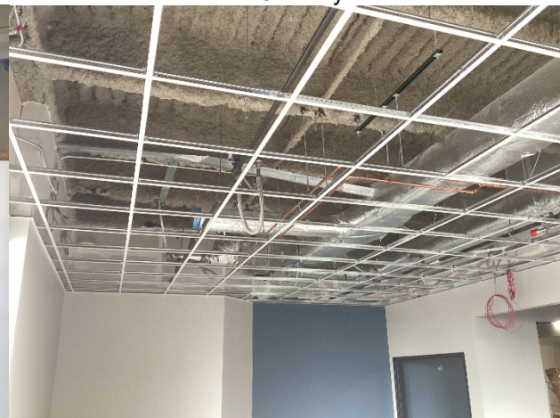
2nd Floor Ceiling Grid Install
