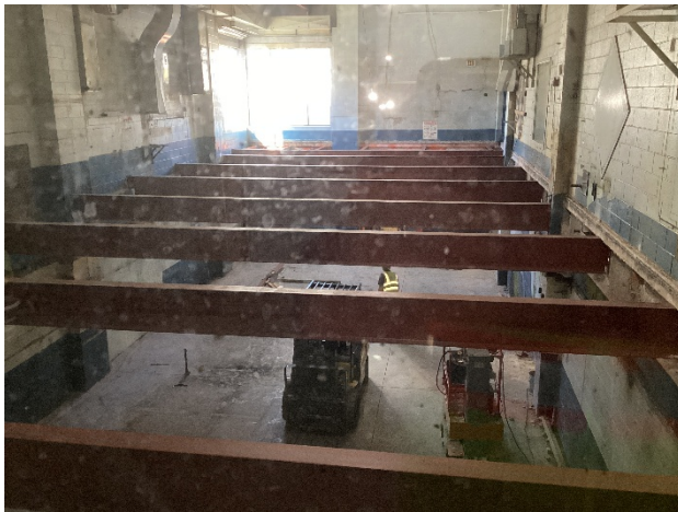
Structural Steel Members Installed
