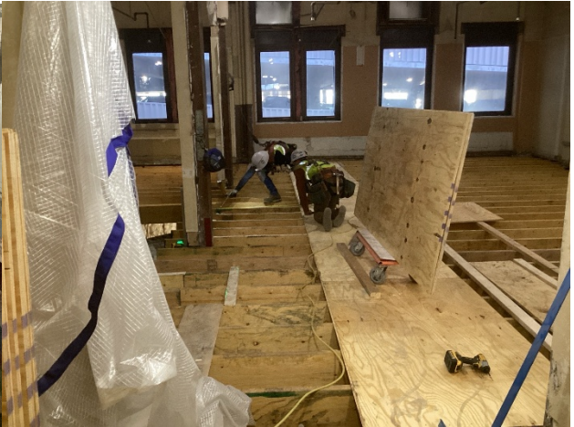
1st Floor Joist System Rebuild
