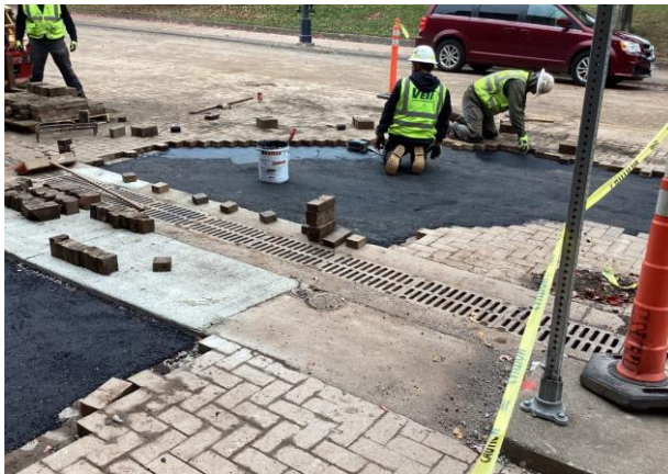
Exterior Water Line Installation
