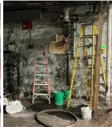
Interior New Water Service
