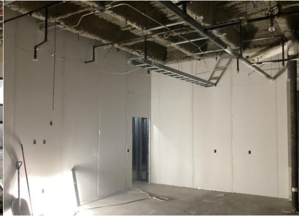
Drywall Installation
