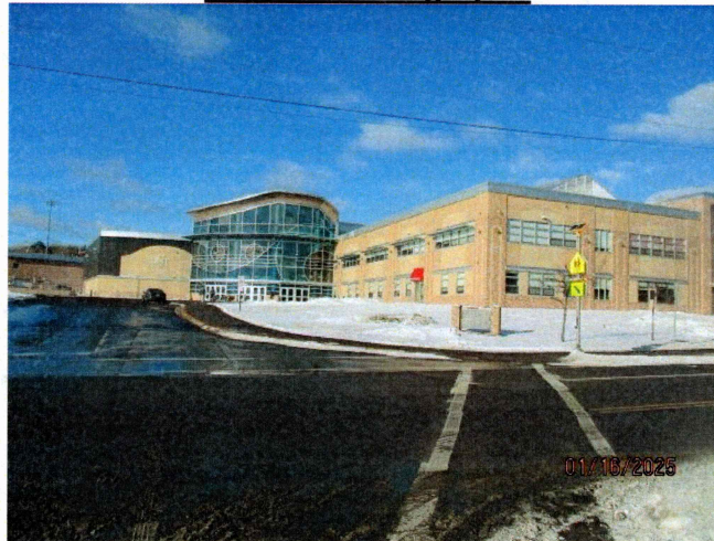
Looking At Subject Improvement From N 40 th Ave E
