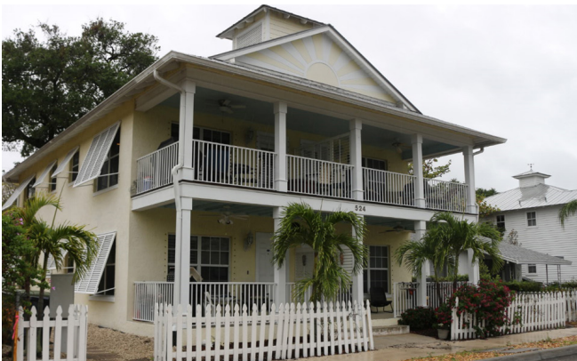
A 2-STORY PORCH ON AN APARTMENT BUILDING.
