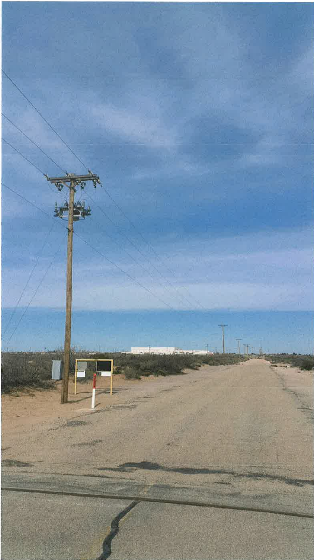
View of major utilities on LTV Rd. not disclosed on Vacation of Right-of-Way Application, including three-phase industrial power and buried fiber optic cable
