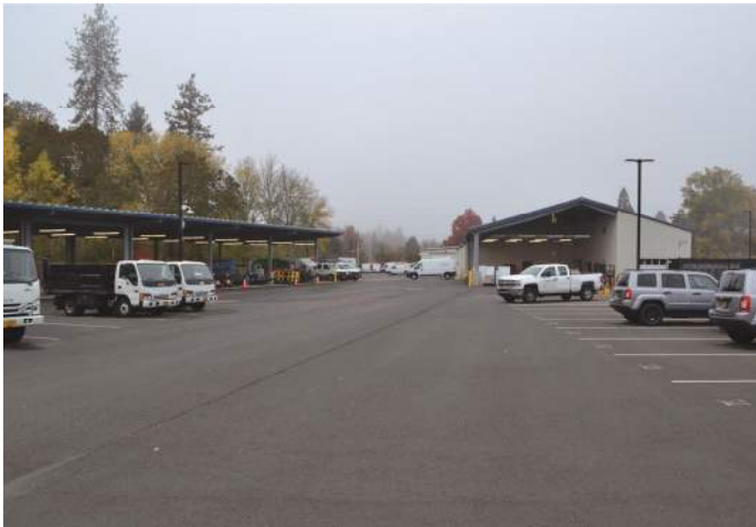
Fig 15. Beaverton Maintenance Yard
