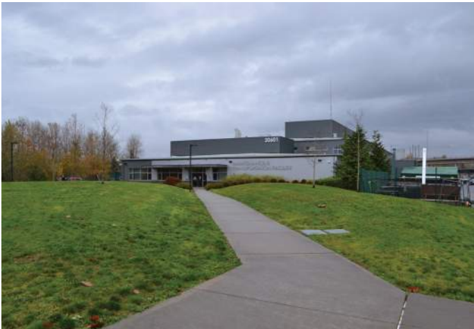
Fig 29. ESD Maintenance & Transportation Facility
