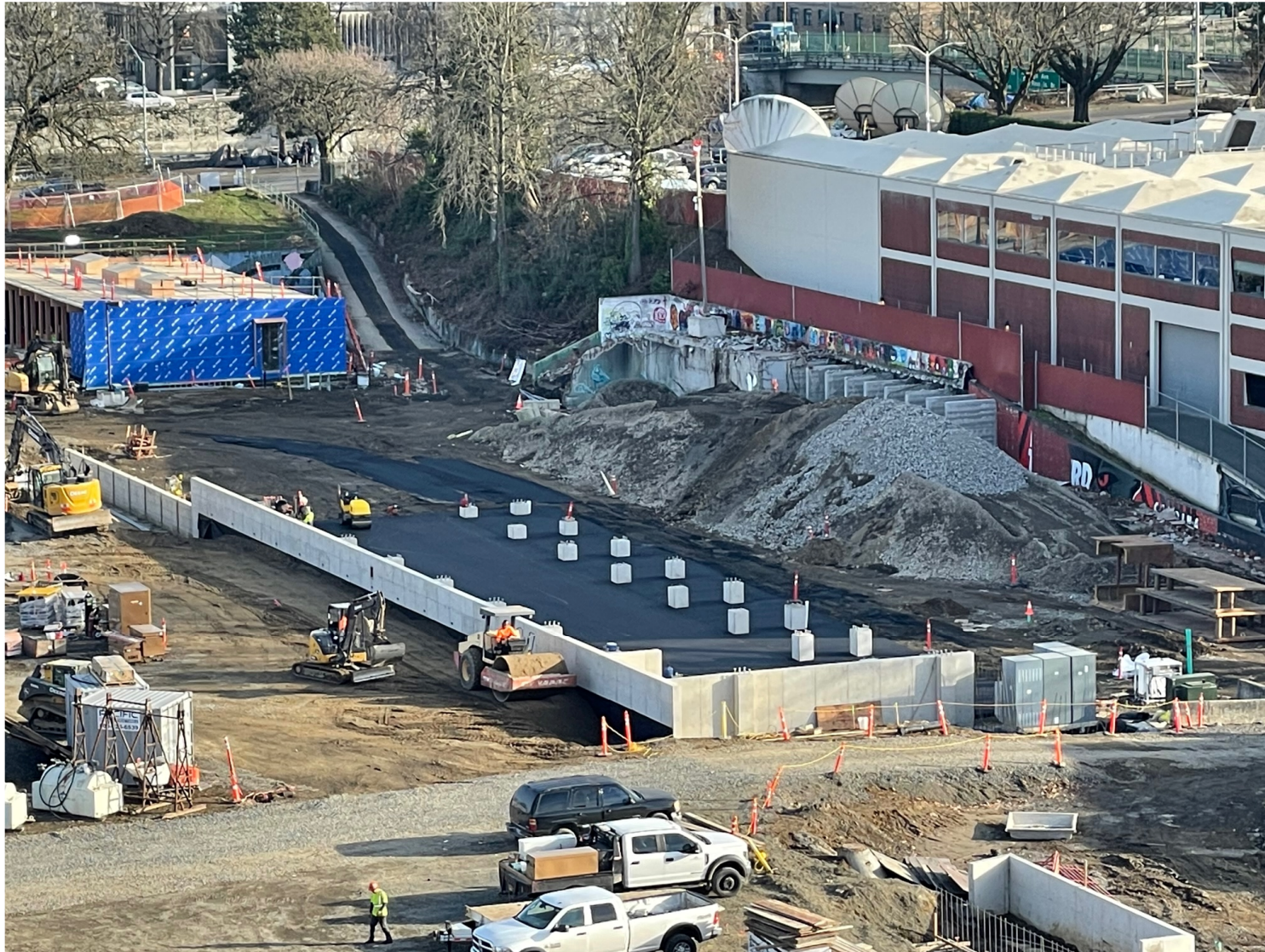
Phase 2 Site Work
