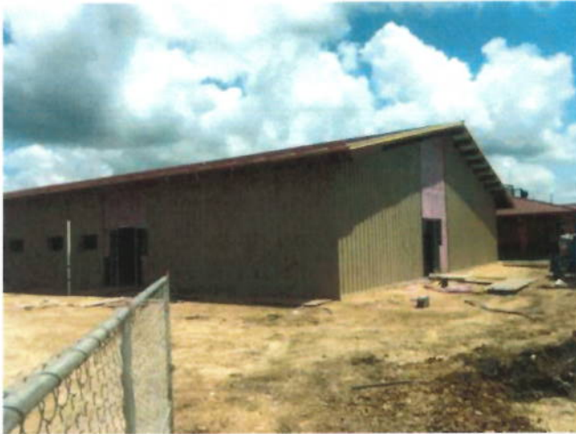
7. Installation of metal wall panels
