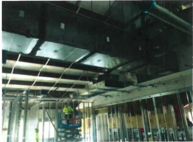
10. Interior partition framing
