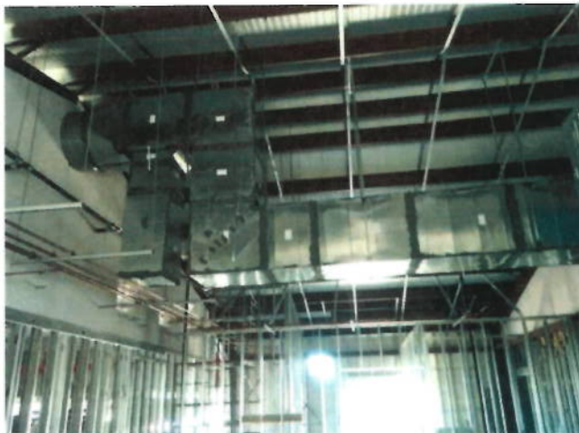
5. Installation of HVAC duct
