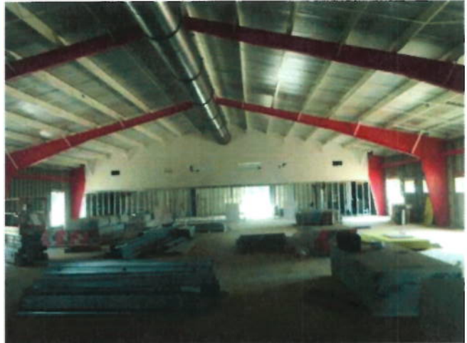
8. Partition framing and drywall at interior
