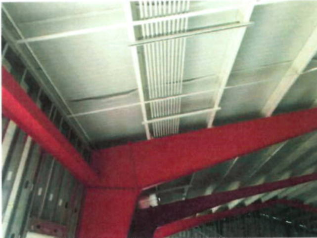
1. Painting of interior beams and MEP systems
