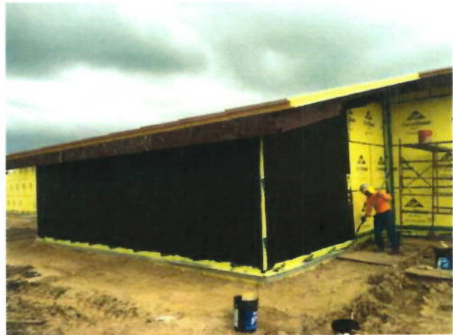
2. Exterior partition air barrier
