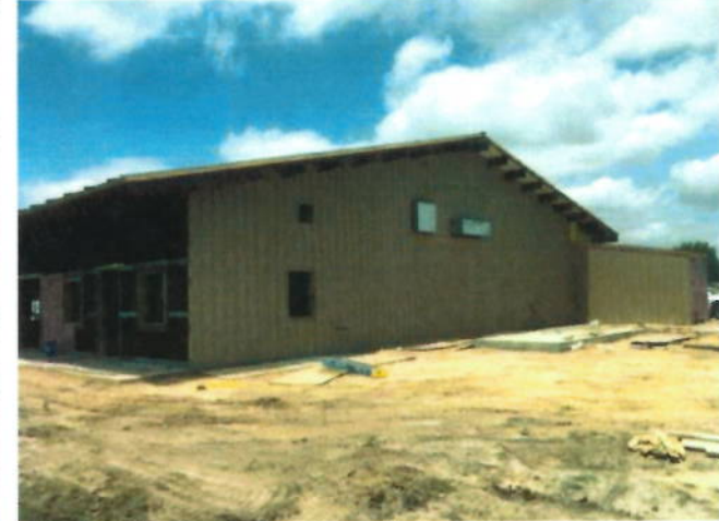
6. Installation of metal panels
