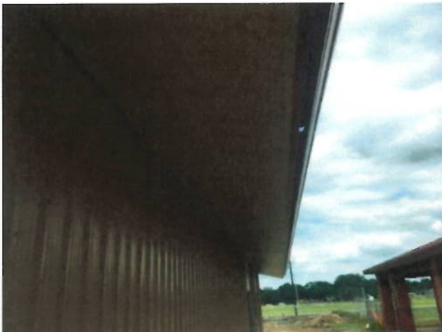
9. Soffit panel installation
