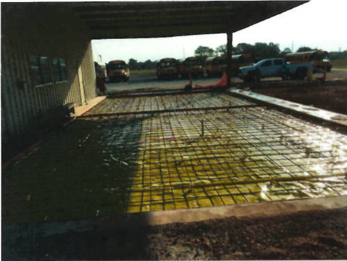
1. Concrete prep at existing open bay
