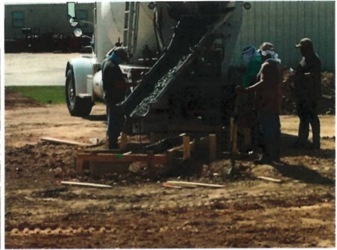
2. Concrete beams for fuel storage tank
