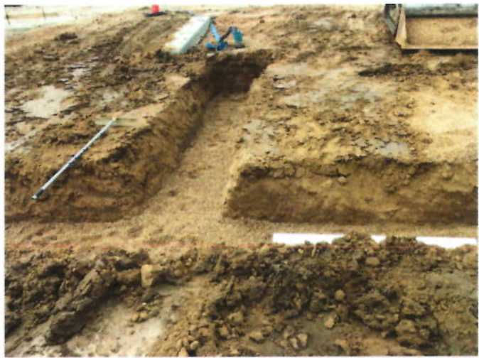
4. Excavation for underground fuel piping
