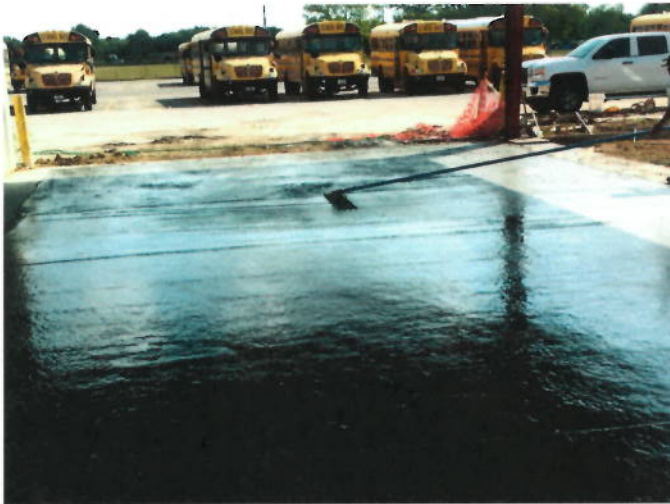
3. Concrete placement at existing open bay
