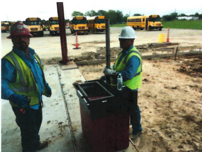
5. Fuel dispenser sump prep
