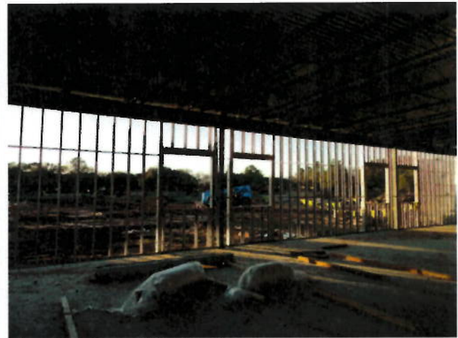
4. Exterior partition framing
