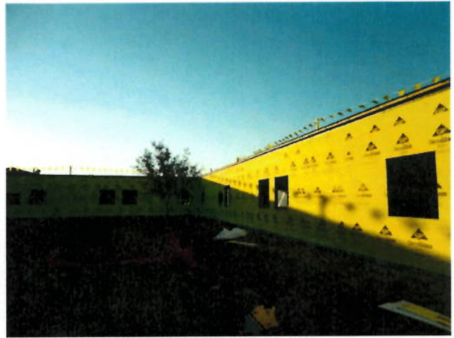
2. Exterior sheathing at south elevation
