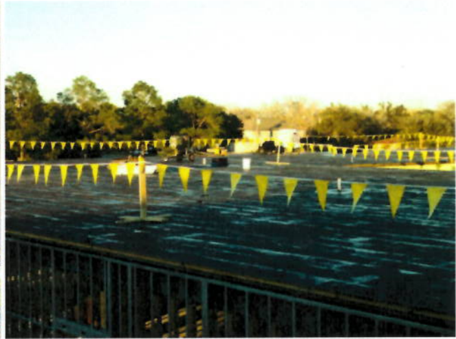
8. Classroom addition roof system installation
