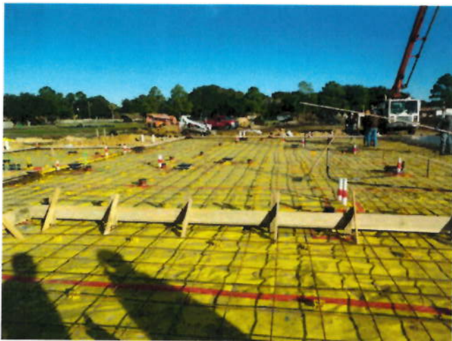
5. Kitchen area plumbing and electrical
