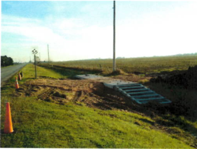
1. Driveway box culverts and safety end treatments
