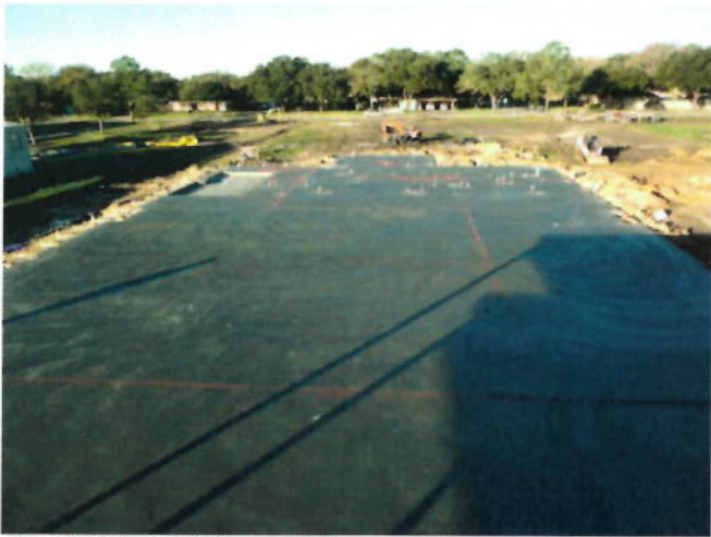
7. Cafeteria slab on grade
