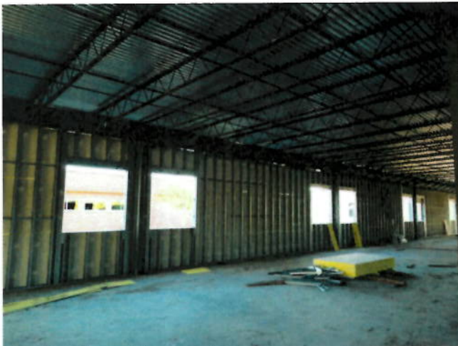
3. Exterior partition framing
