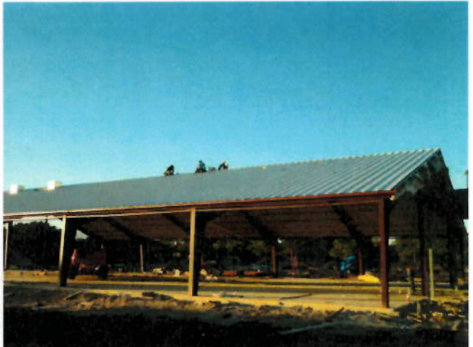
6. Cafeteria metal roofing
