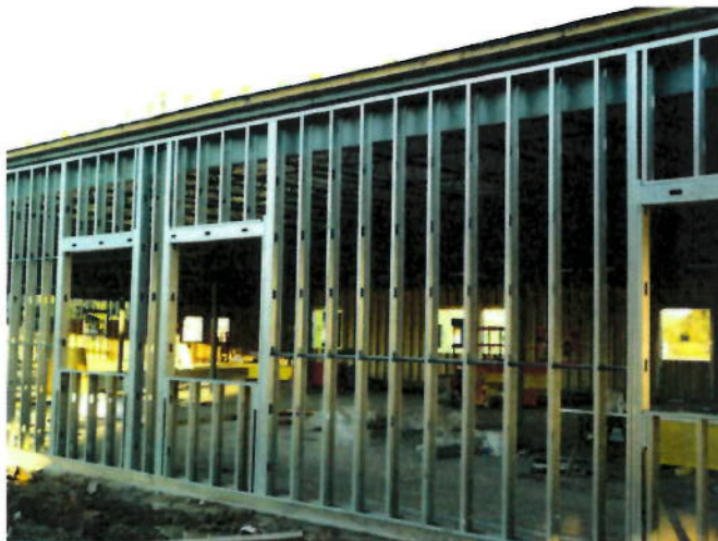
11. Exterior partition framing
