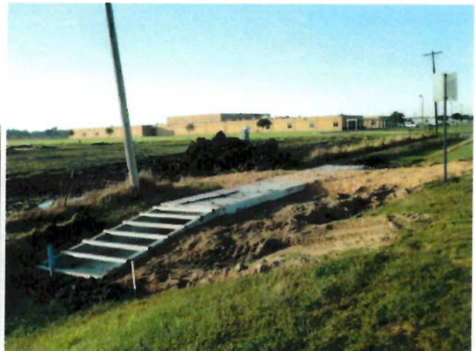
2. Driveway box culverts and safety end treatments
