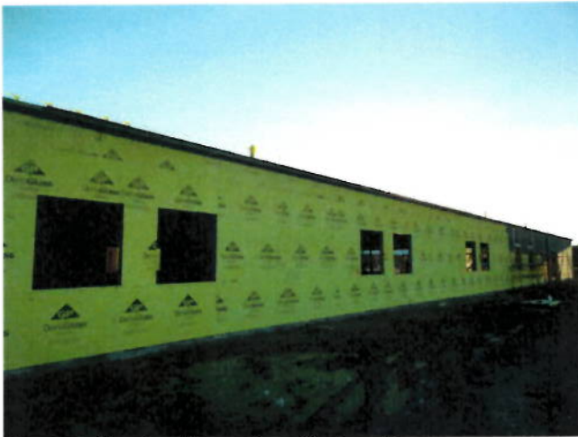
1. Exterior sheathing at south elevation
