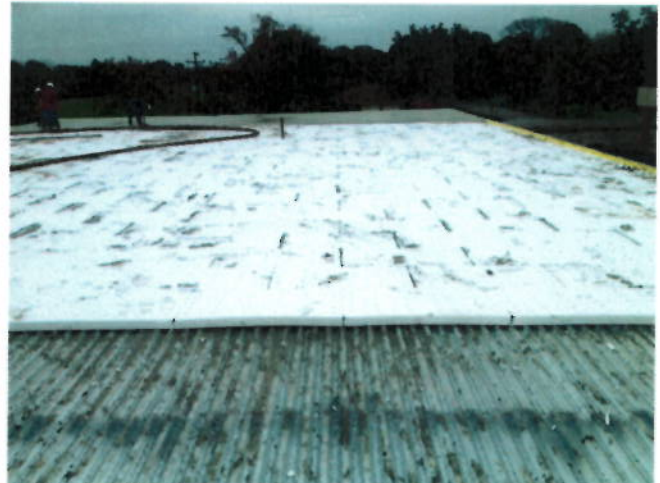
10. Lightweight roof deck installation
