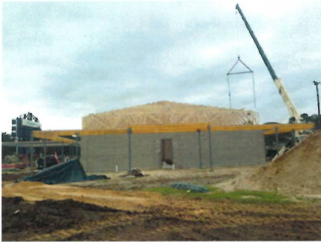
1. Main roof wood truss east elevations
