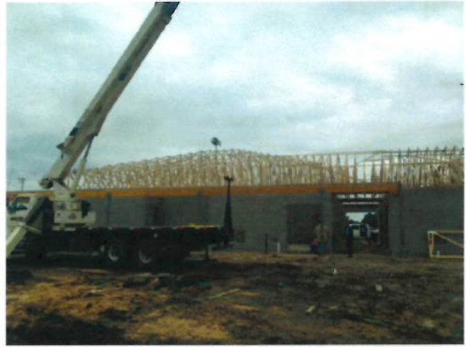
2. Main truss roof system at home side
