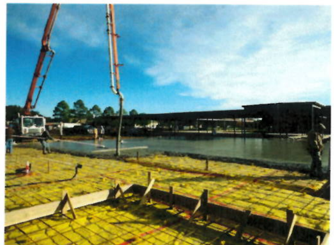
4. Concrete pumping equipment
