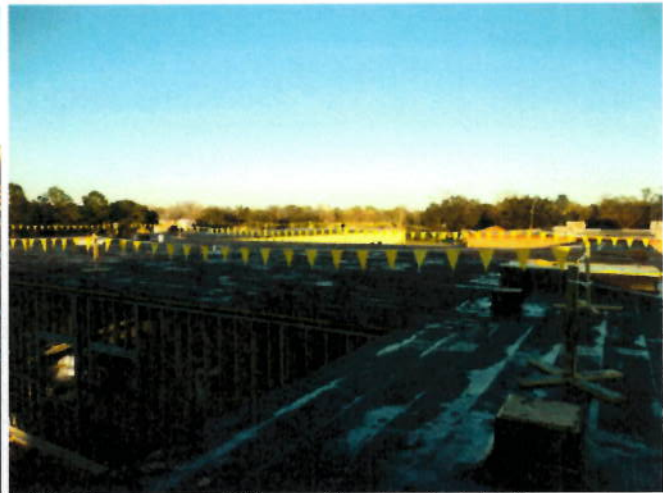
10. Classroom addition roof system installation
