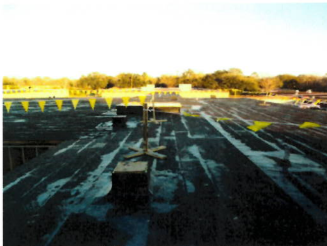
9. Classroom addition roof system installation
