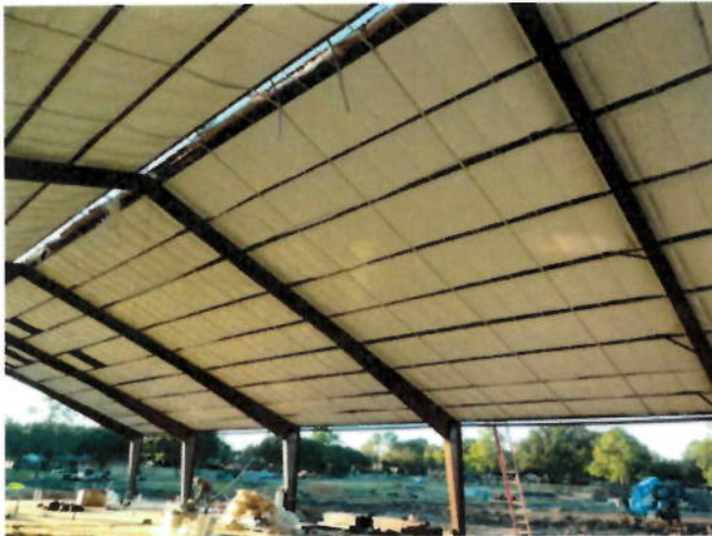
7. Cafeteria PEMB roof insulation
