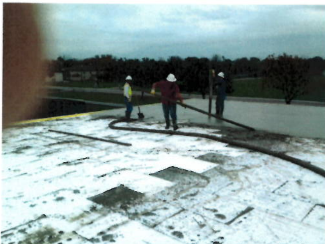
11. Vermiculite roof deck application
