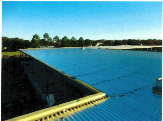
8. Metal roof deck at classroom addition
