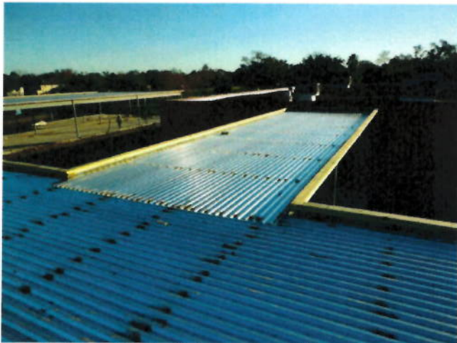
9. Metal roof deck at classroom addition
